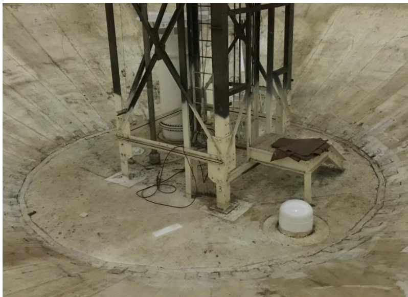
Figure 2-15 – Base of Tank 5 Tower
