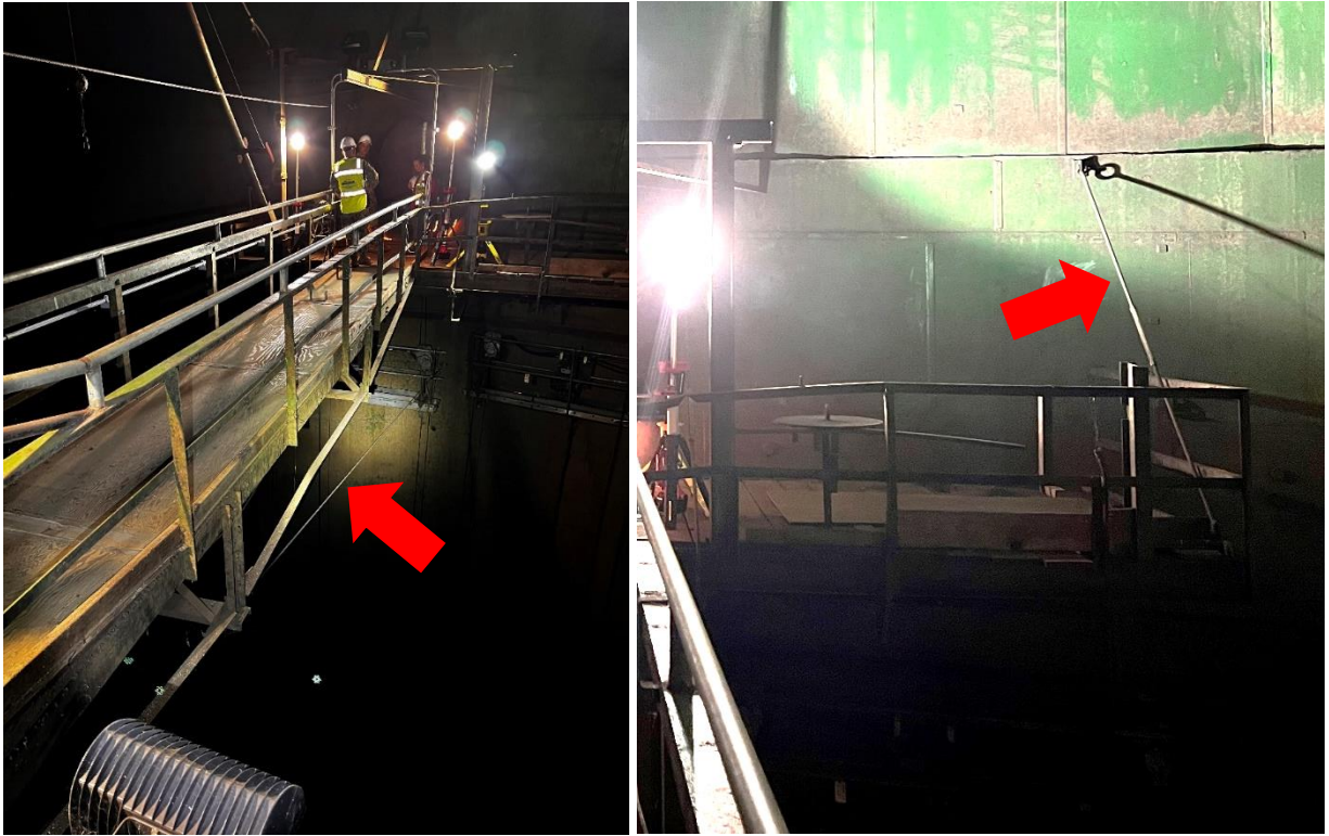
Figure 2-18 – Tank Tower Access Bridge (Left) and Entry Platform (Right)
