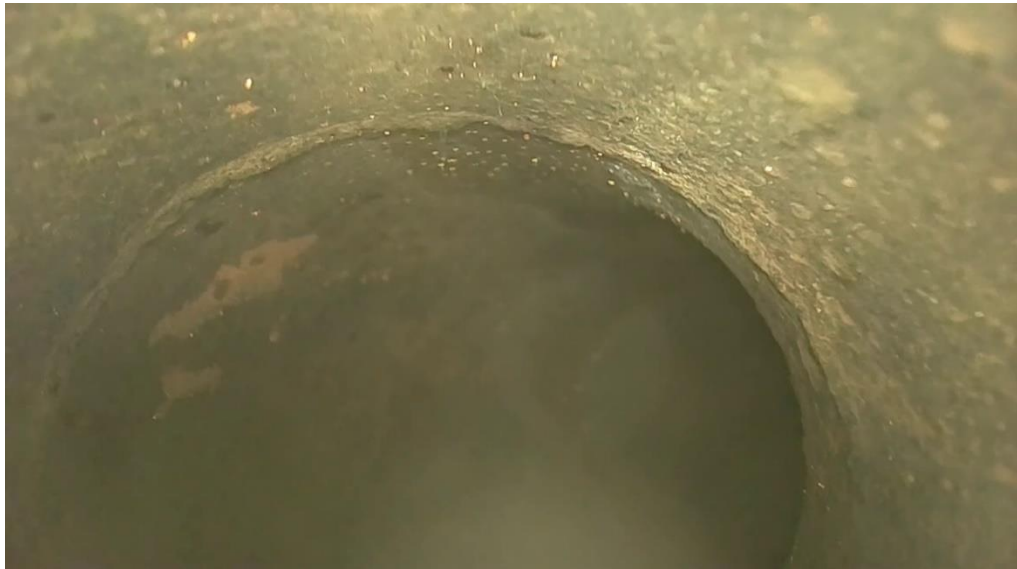
C.15 Third elbow after pipe spool (from entry point A)
