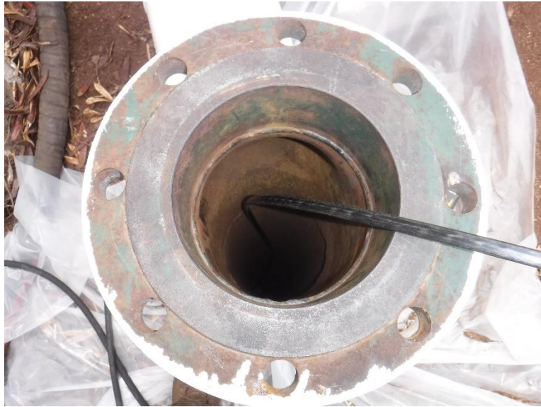
C.4 Borescope inspection entry point A (flange removed)
