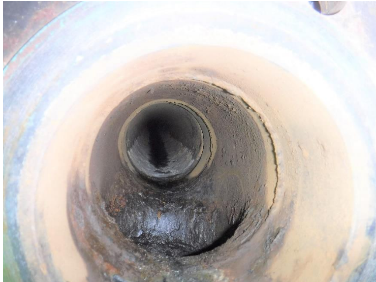
C.25 Entry Flange B (Interior of pipe after cleaning)
