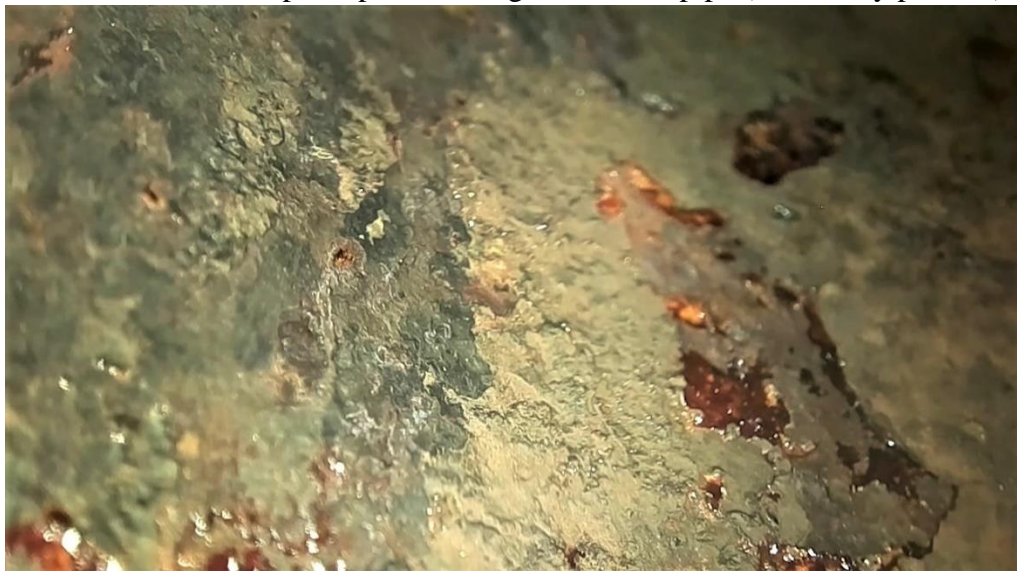
C.12 Borescope inspection image bottom of pipe (from entry point A)
