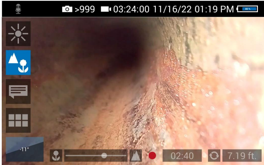
C.31 Boreoscope inspection image, side of pipe (from entry point B)
