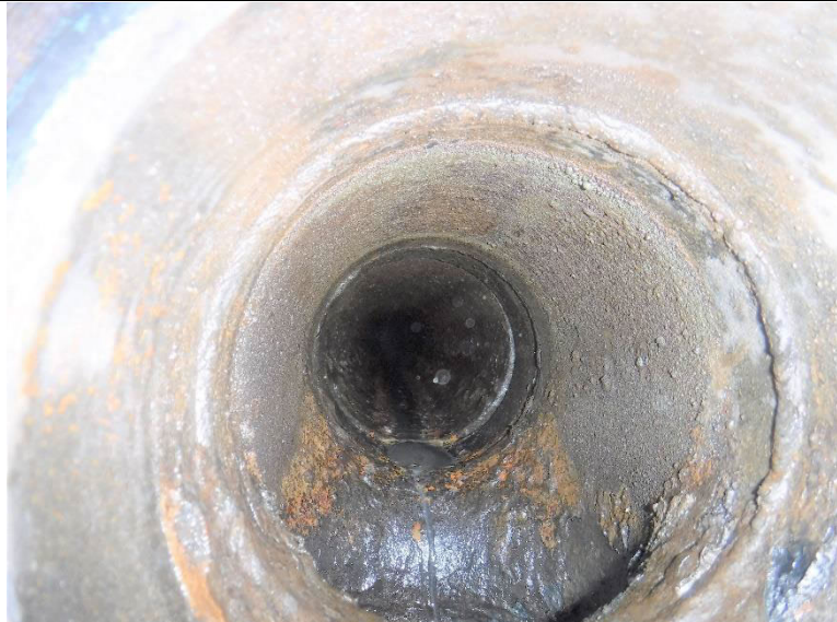
C.21 Entry Flange B (Interior of pipe before cleaning)
