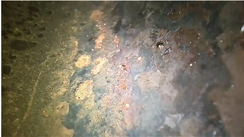
C.11 Borescope inspection image bottom of pipe (from entry point A)
