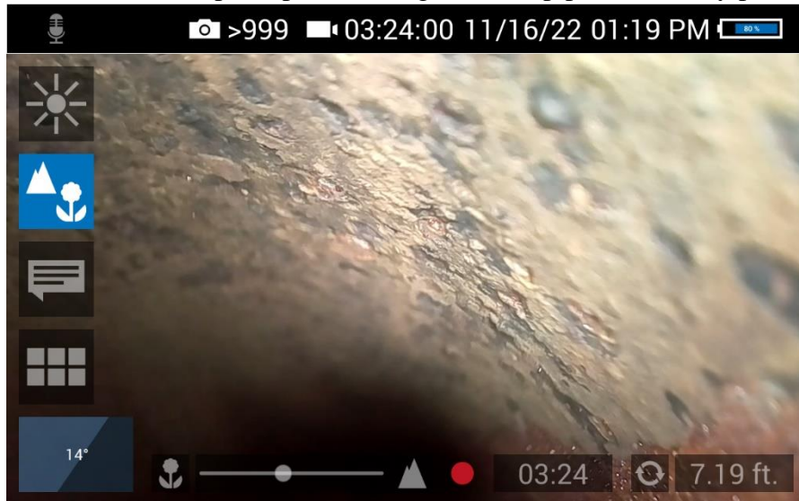
C.32 Boreoscope inspection image, top of pipe (from entry point B)
