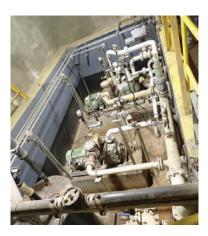
Figure 1: Main Containment Sump for Fuel Oil Reclamation
