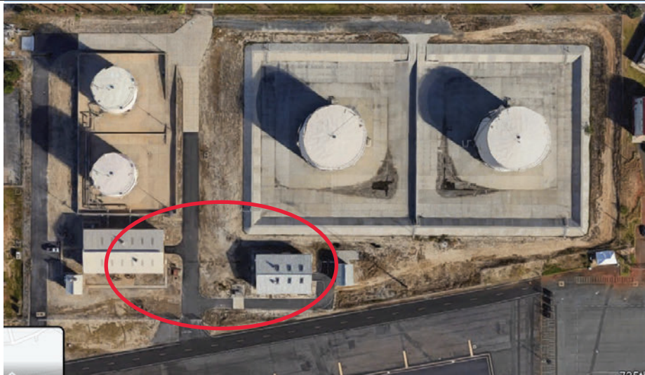
Hickam ASTs and PRT Tanks
