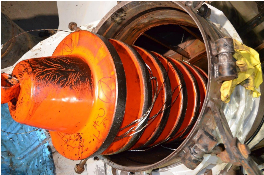
FIGURE 2-2: CLEANING PIG AFTER IT HAS BEEN REMOVED FROM THE RECEIVER
