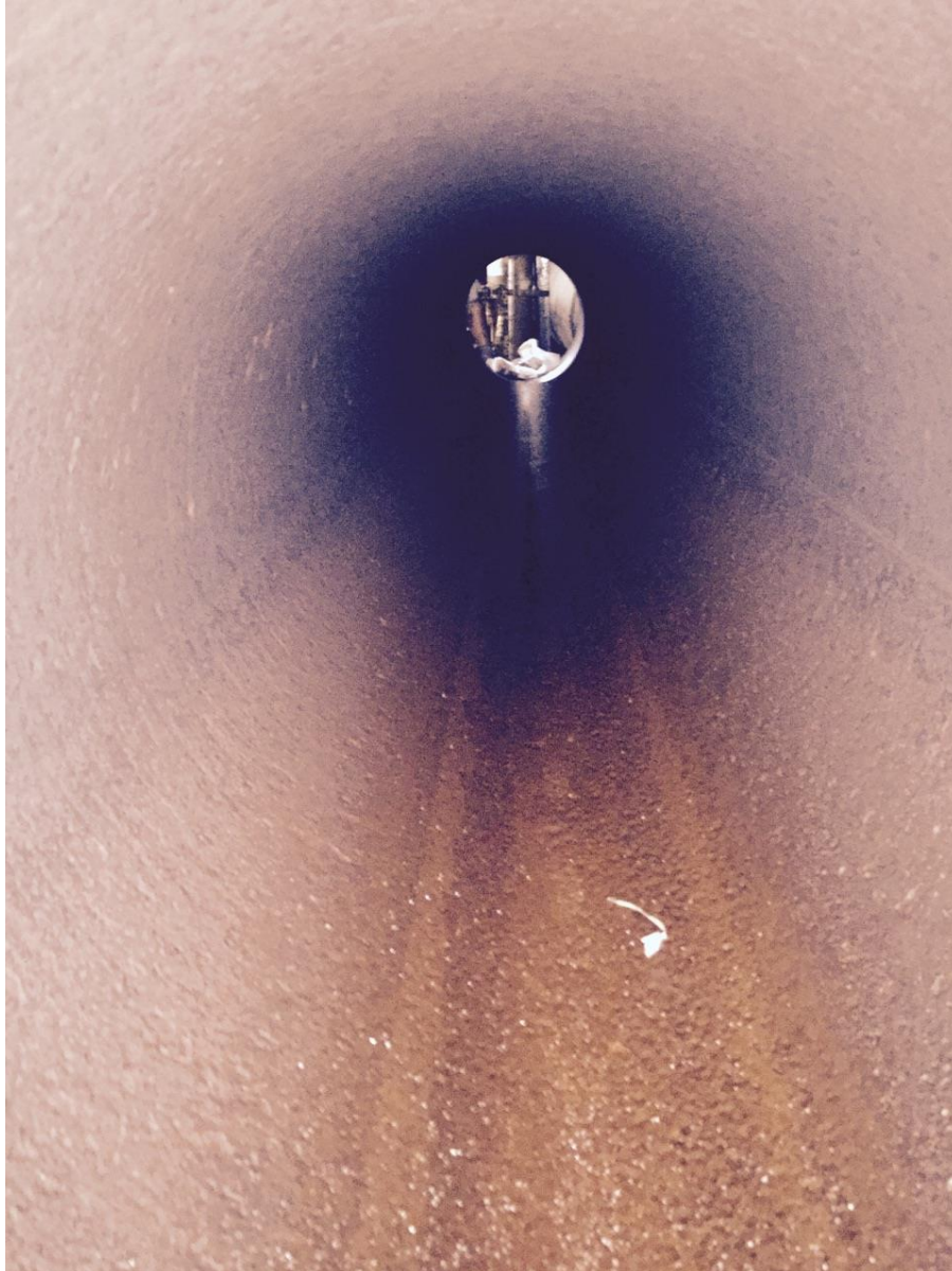
FIGURE 2-3: TYPICAL CLEANED SECTION OF PIPING AFTER PIGGING
