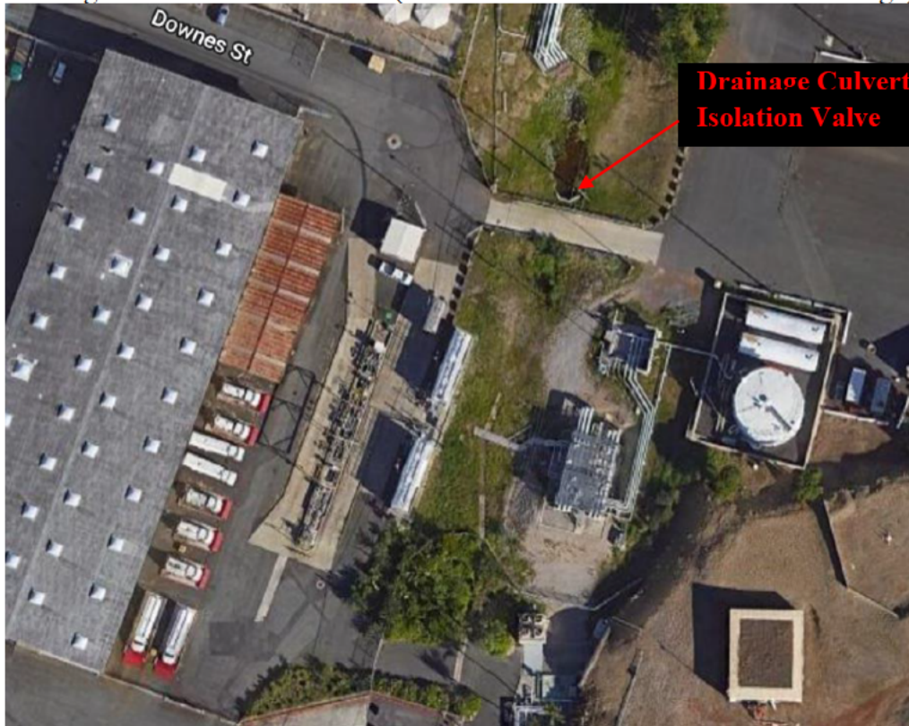
Drainage Culvert Isolation Valve (Aerial View and Ground View from Bridge):
