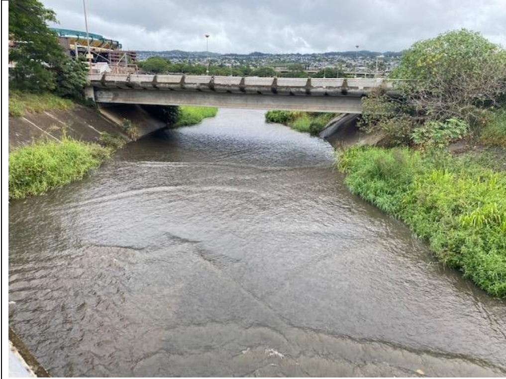
Photograph # 1: Downstream Site #1 looking upstream.
