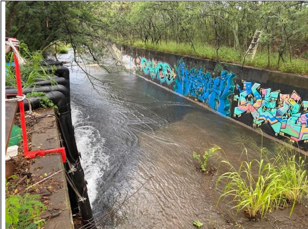
Photograph # 2: Discharge Site looking downstream.
