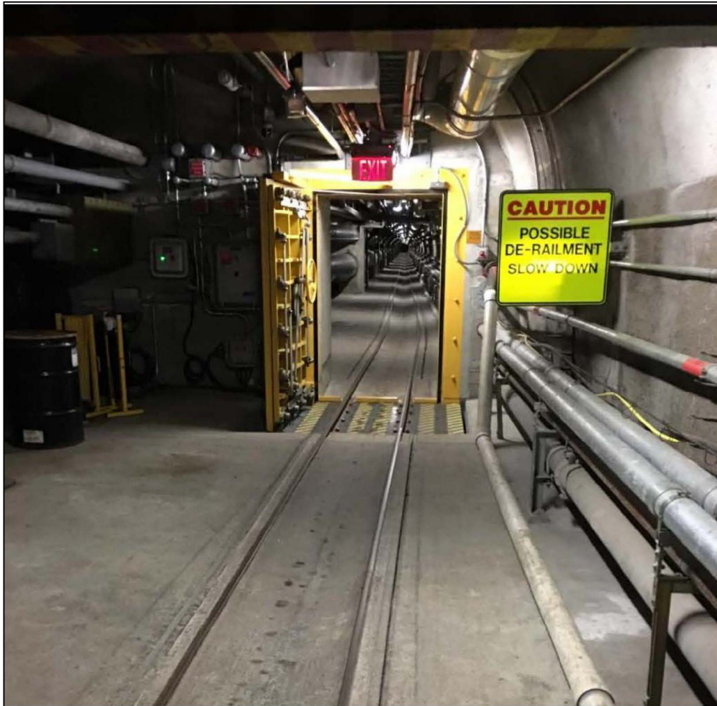
Figure 4.1: Emergency Oil Pressure Door
