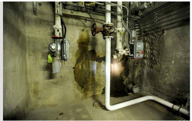
COURTESY U.S. NAVY / SENIOR CHIEF MASS COMMUNICATIONS SPECIALIST MICHAEL B. LEWIS A close-up of the wet spot in the concrete below Tank 5 at the Red Hill Underground Fuel Storage Facility. The wet material matched the jet fuel that was emptied from Tank 5. The floor drain in lower right captures spilled material before it enters the environment.
