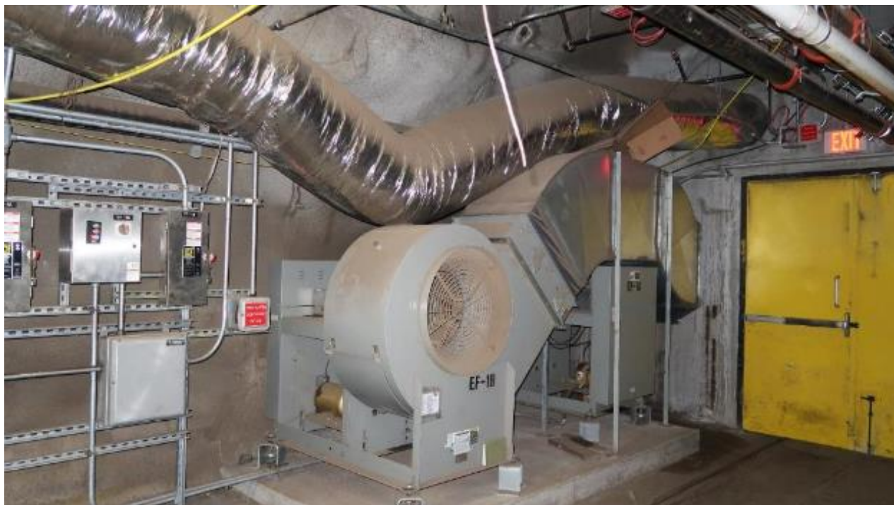
Existing Upper Tunnel Exhaust Fan Note temporary construction venting duct above fan
