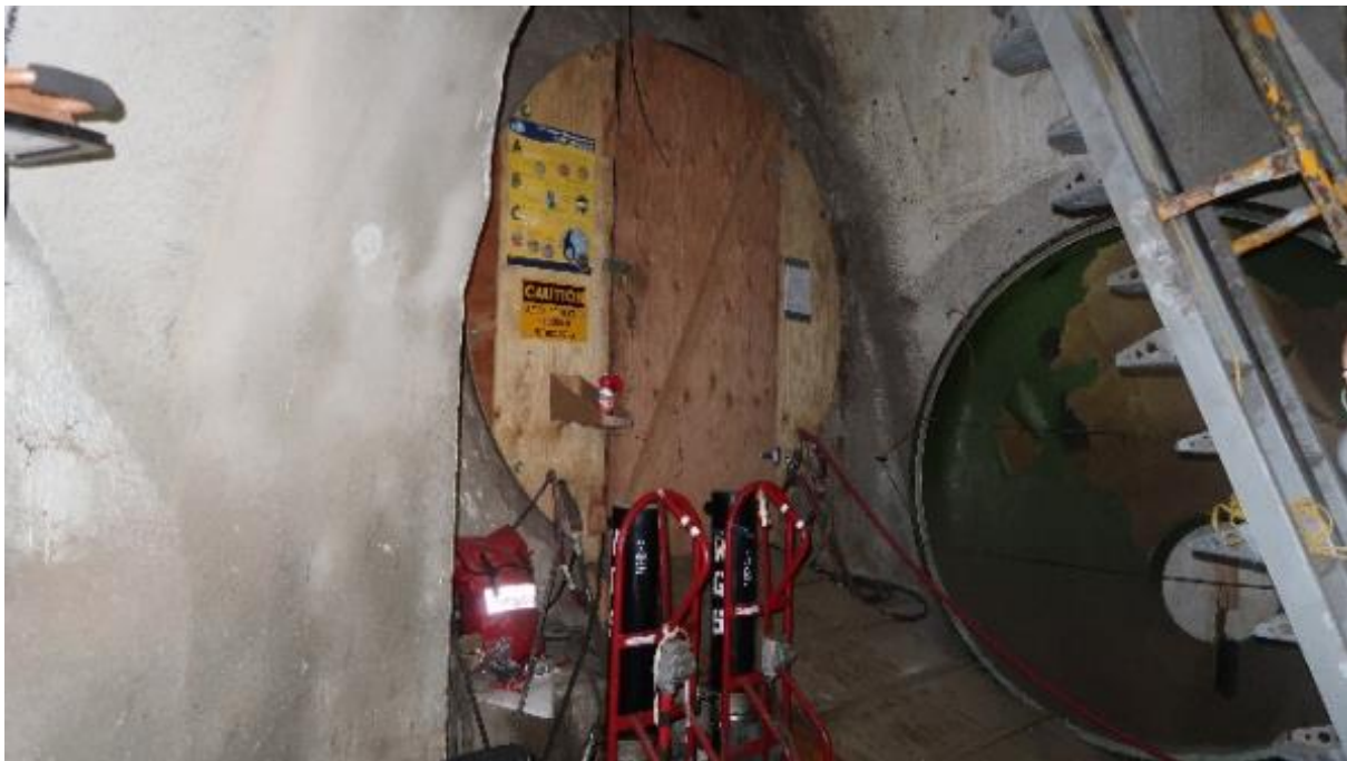
All materials must be loaded through the 8-feet diameter tank manhole
