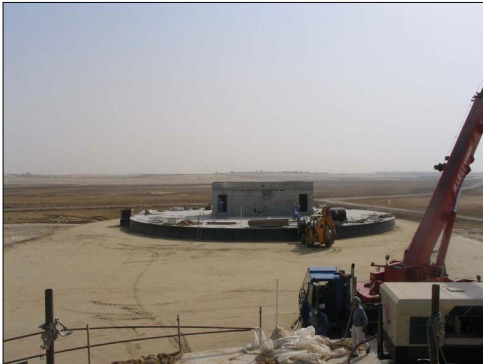
Photograph 2.2-12 Completed underground vertical (cut-and-cover) storage tank.
