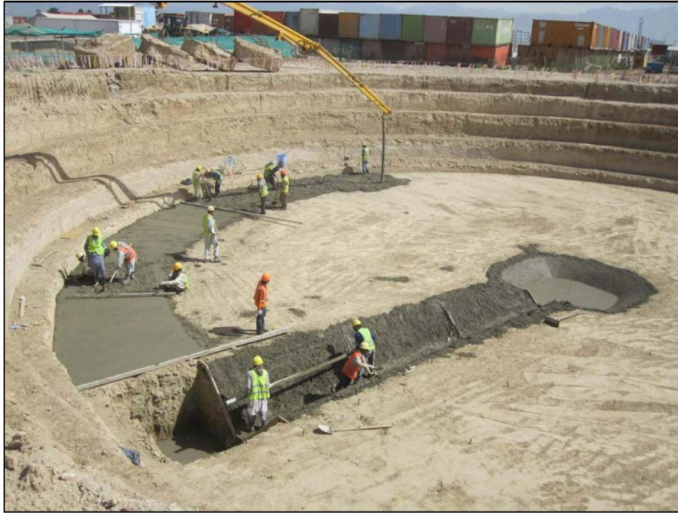
Photograph 2.2-1 Excavation and initial leveling course.
