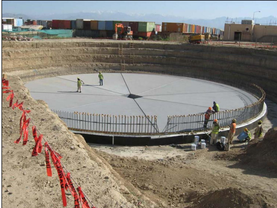
Photograph 2.2-6 Completed foundation slab with radial drainage gutters.
