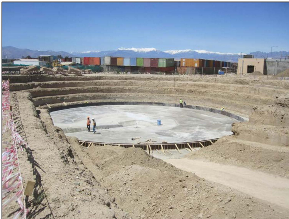
Photograph 2.2-2 Completed leveling course.
