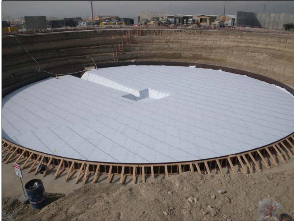
Photograph 2.2-3 Waterproof membrane.
