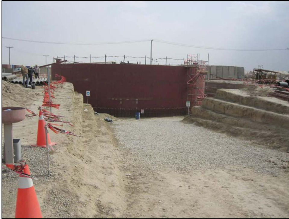
Photograph 2.2-9 Completed welded steel tank.
