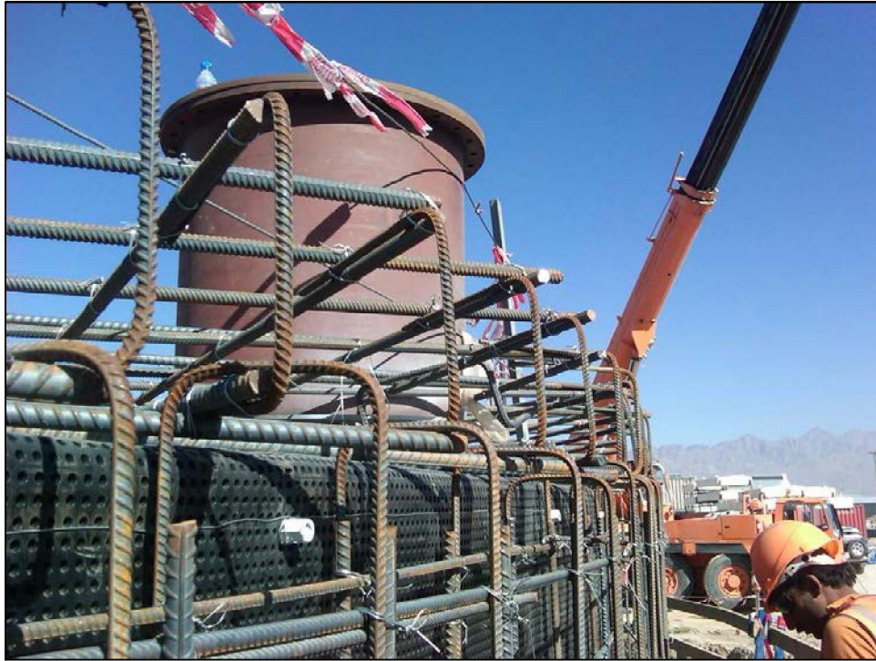
Photograph 2.2-11 Geosynthetic drainage layer (black material with dimples).
