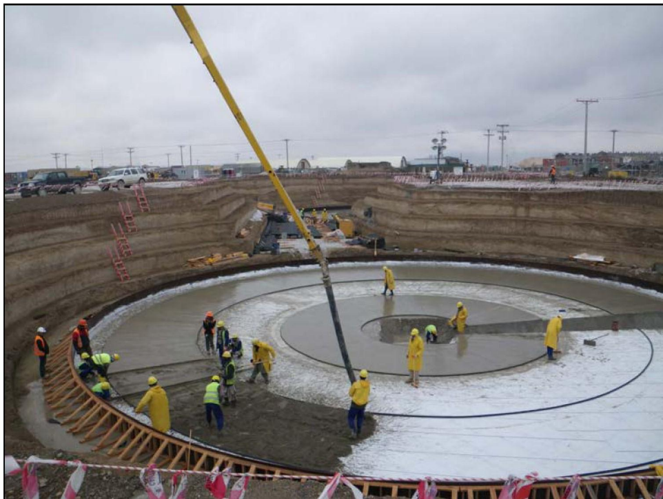
Photograph 2.2-4 Protective grout course.
