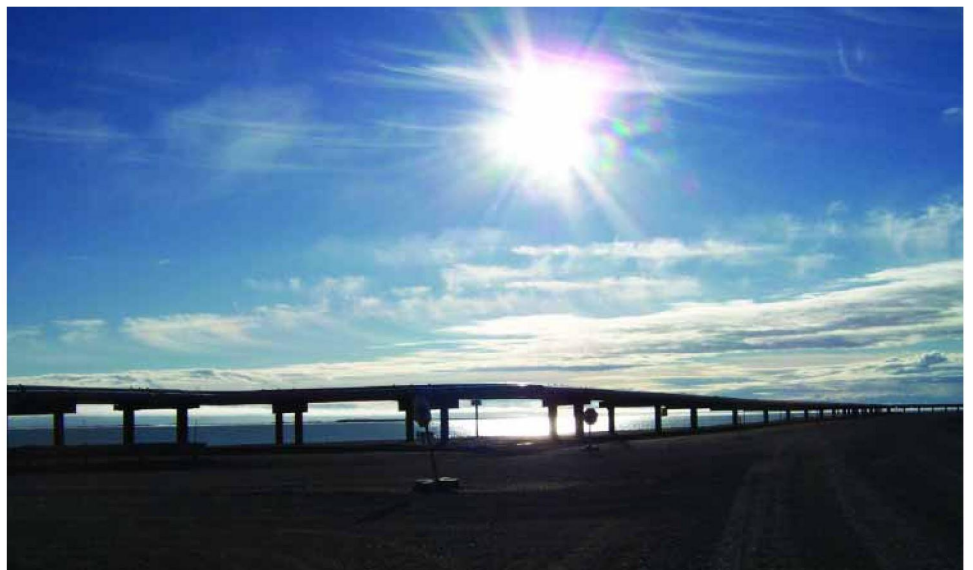
Figure 9. Petroleum transit pipelines at Prudhoe Bay cross 11 miles of eco-sensitive Alaskan tundra. The eastern and western transit lines deliver a total of 400 000 barrels of North Slope crude petroleum to the lower 48 states on a daily basis.
