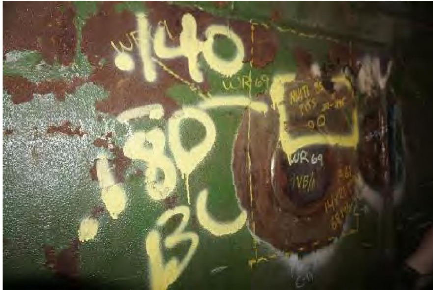
Photo 29: Backside Corrosion around existing patch plates
