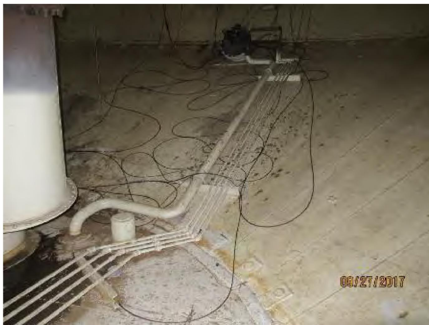
Photo 8: Drain and Sample Lines from new Tank Penetration
