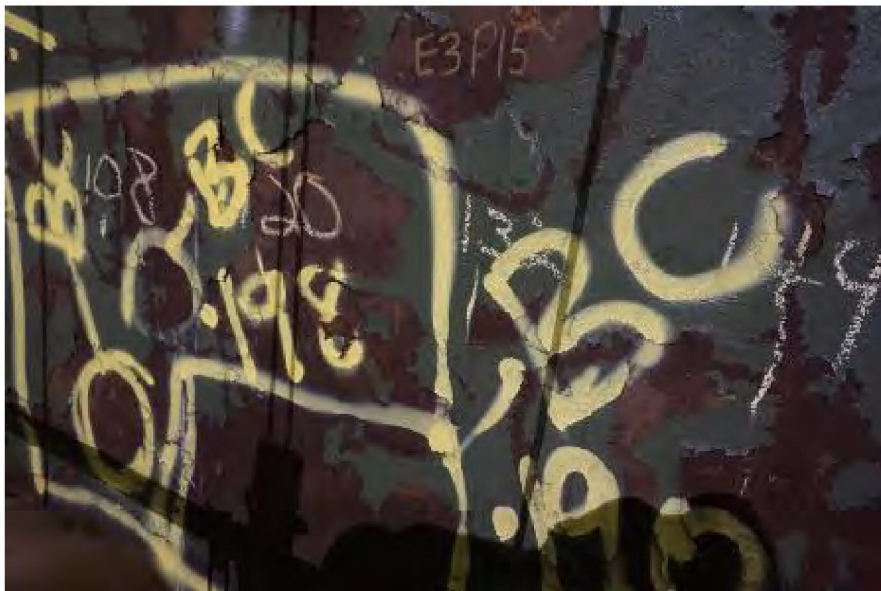
Photo 32: Larger Backside Corrosion Indications in Extension Ring Plates
