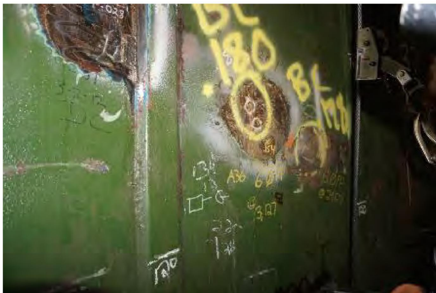
Photo 28: Backside Corrosion on existing ground areas
