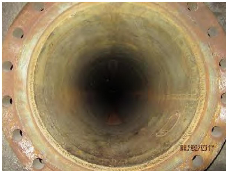
Photo 18: 32-inch pipe with Insert Patch Plate
