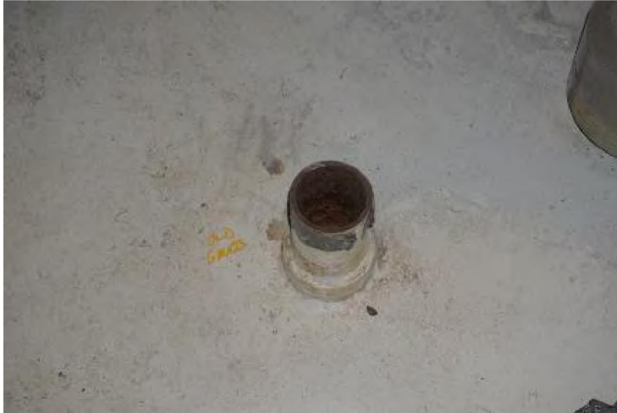
Photo 11: Old stilling well still welded to floor
