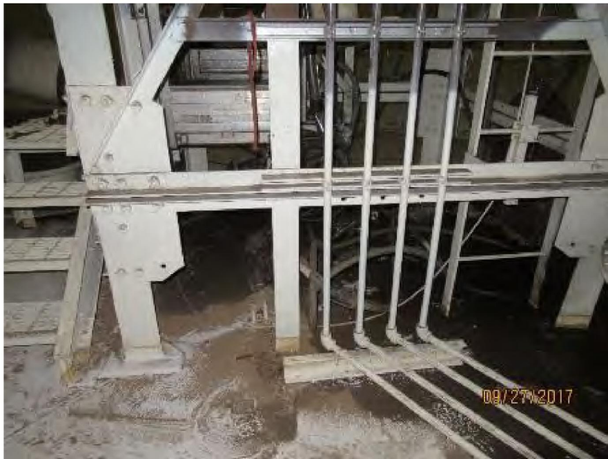
Photo 10: Sample Lines (Note: Supports not seal welded to tank floor).
