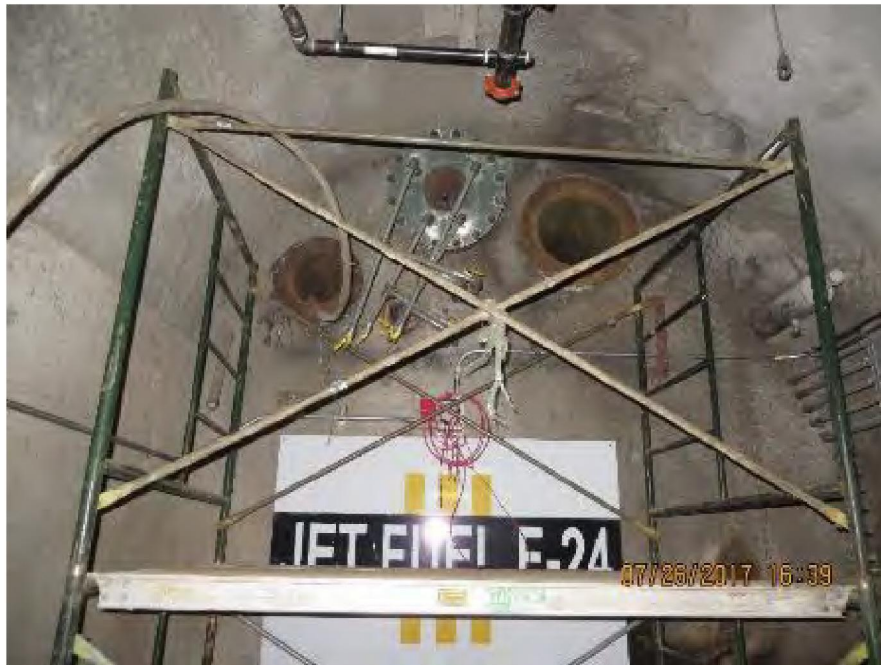
Photo 15: Lower Tunnel Pipe Penetrations
