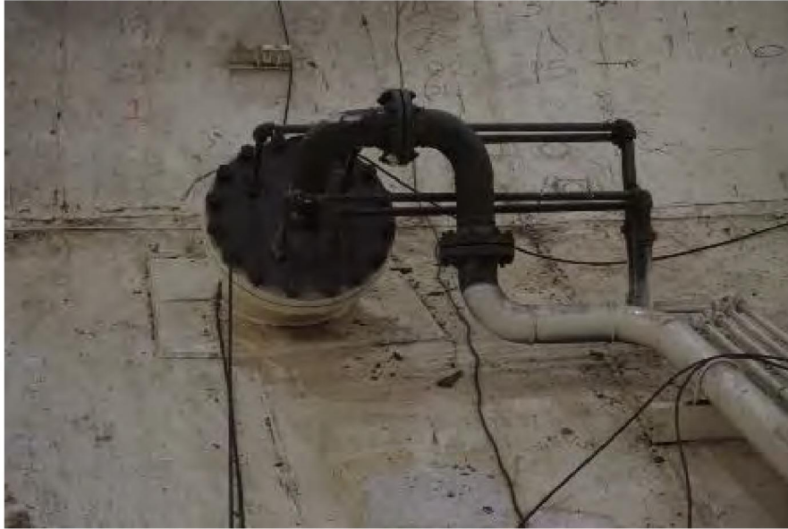
Photo 9: Tank Drain and Sample Lines
