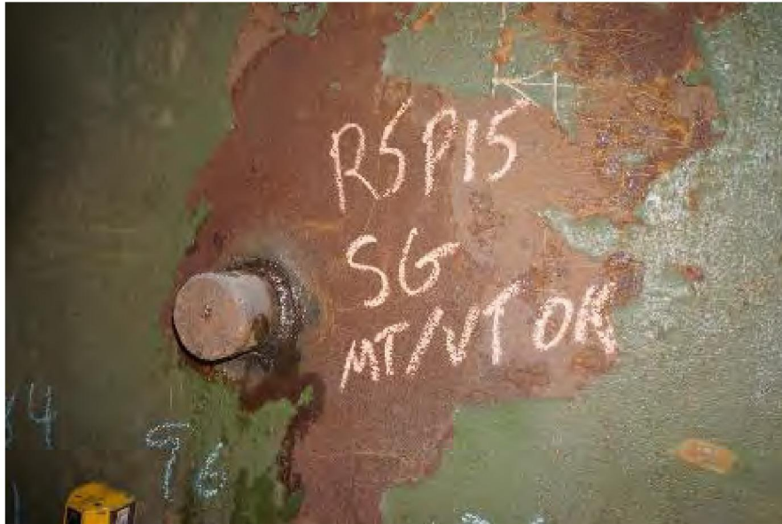
Photo 27: Barrel Strain Gauge Pipe Cap
