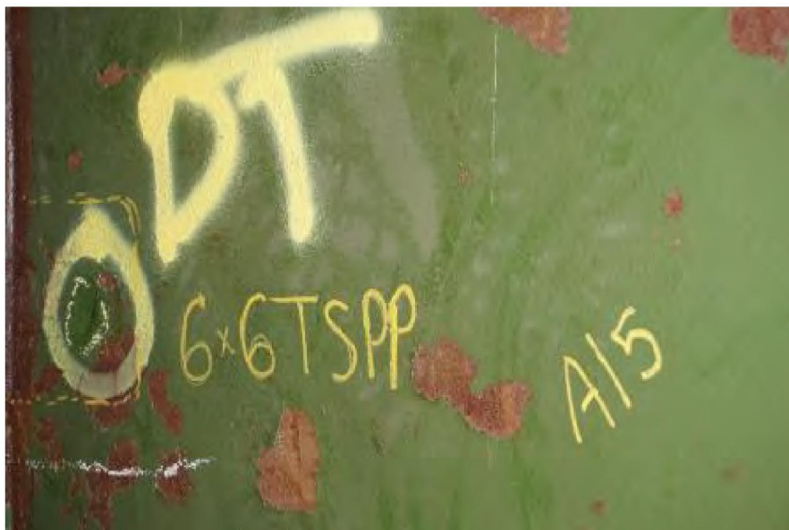
Photo 34: Dent requiring repair in A Course
