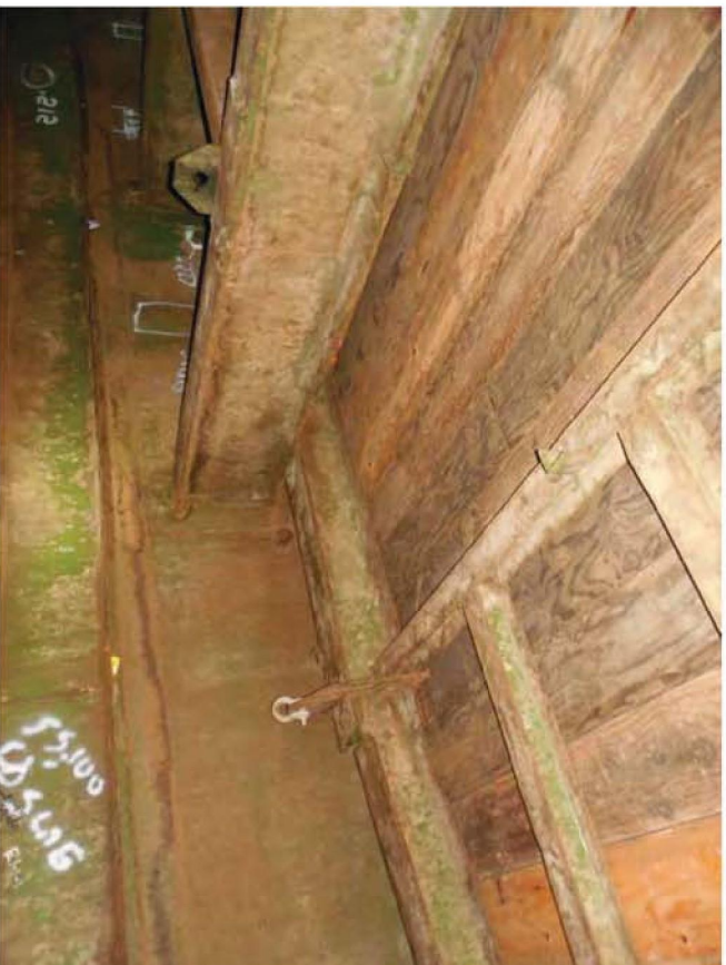
Photo 37: Tank #17 framing – entrance framing
