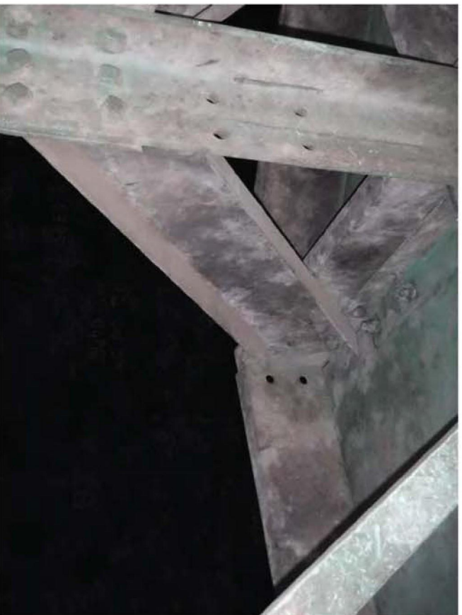
Photo 12: Tank #17 framing at walkway platform level
