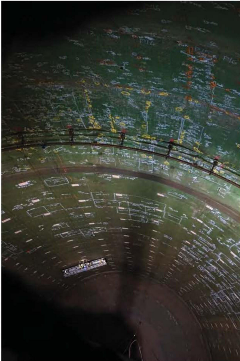
Photo 15: Tank wall from upper dome to lower dome
