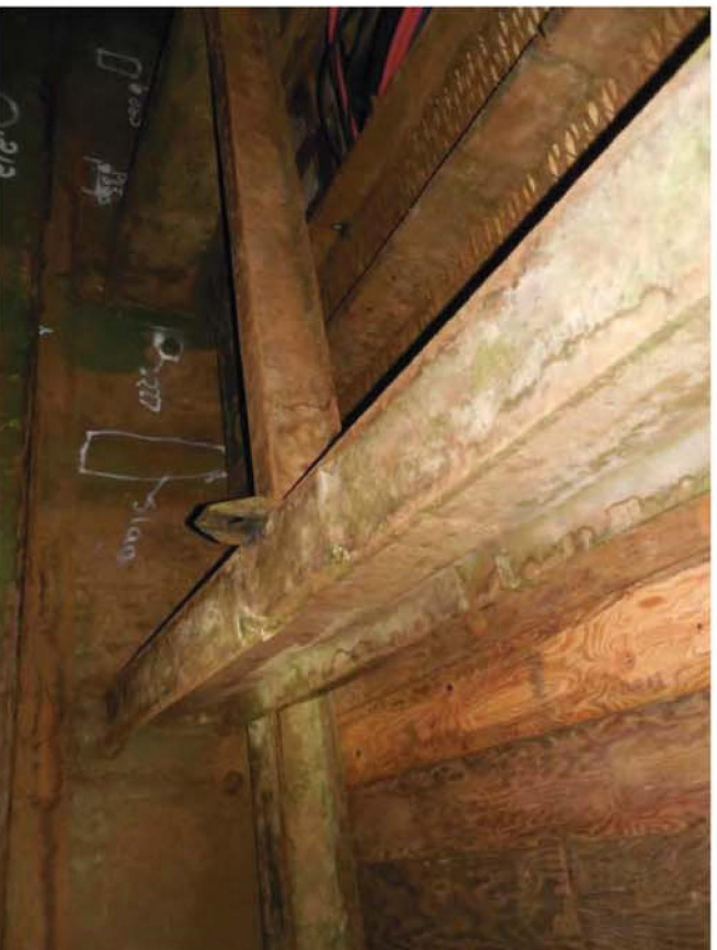
Photo 38: Tank #17 framing – entrance framing
