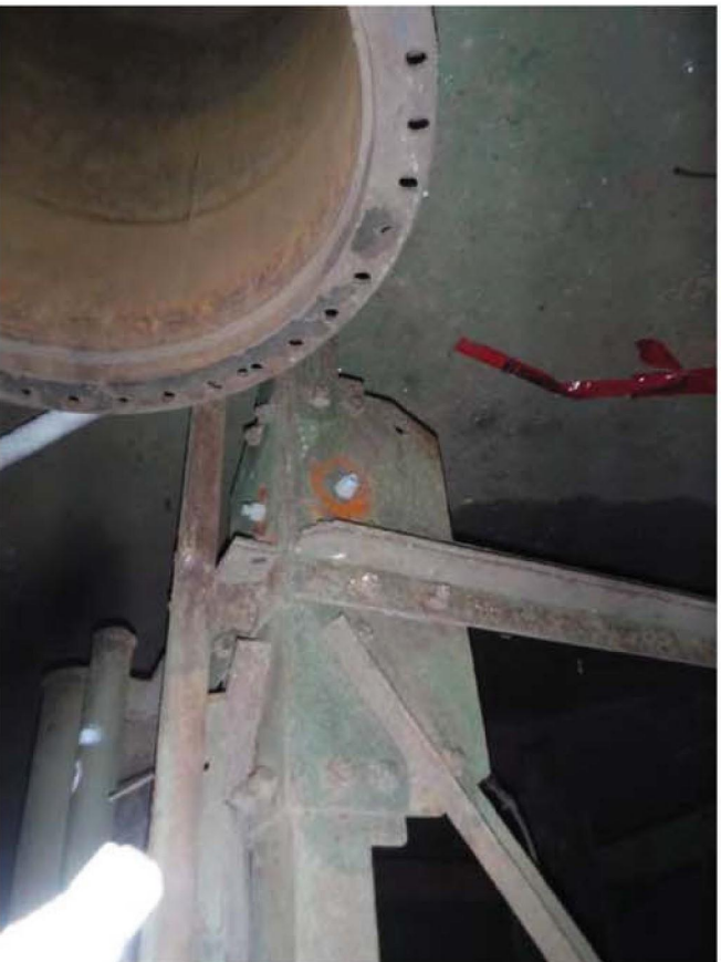
Photo 7: Tank #17 closeup view of tower leg support
