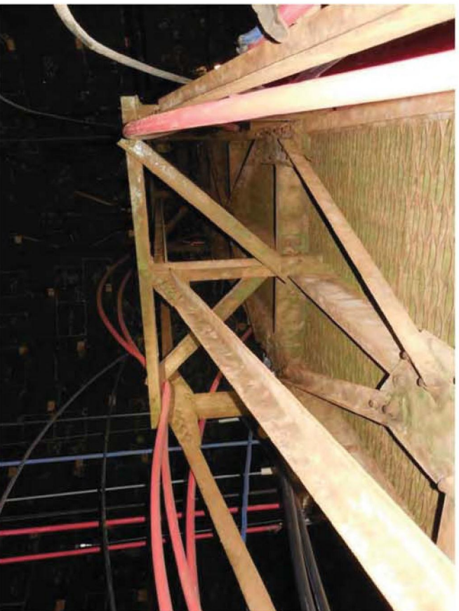
Photo 42: Tank #17 framing – Walkway framing
