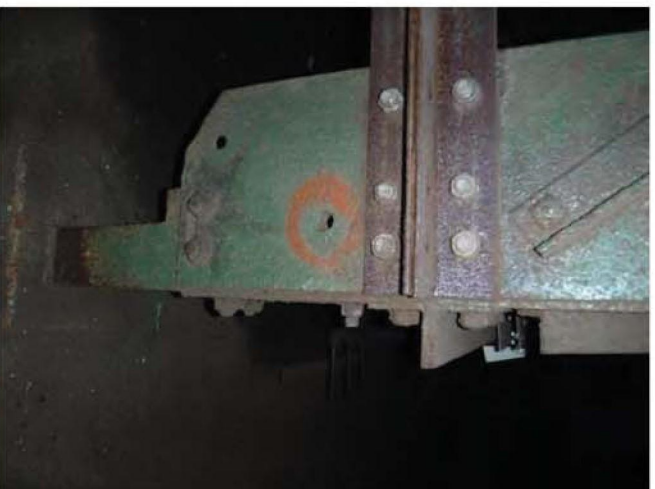
Photo 10: Tank #17 Base tower leg view
