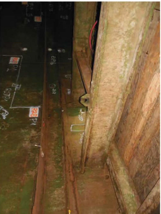
Photo 33: Tank #17 framing – entrance framing
