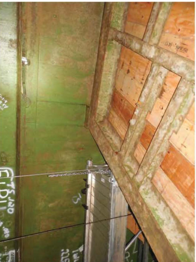
Photo 35: Tank #17 framing – entrance framing
