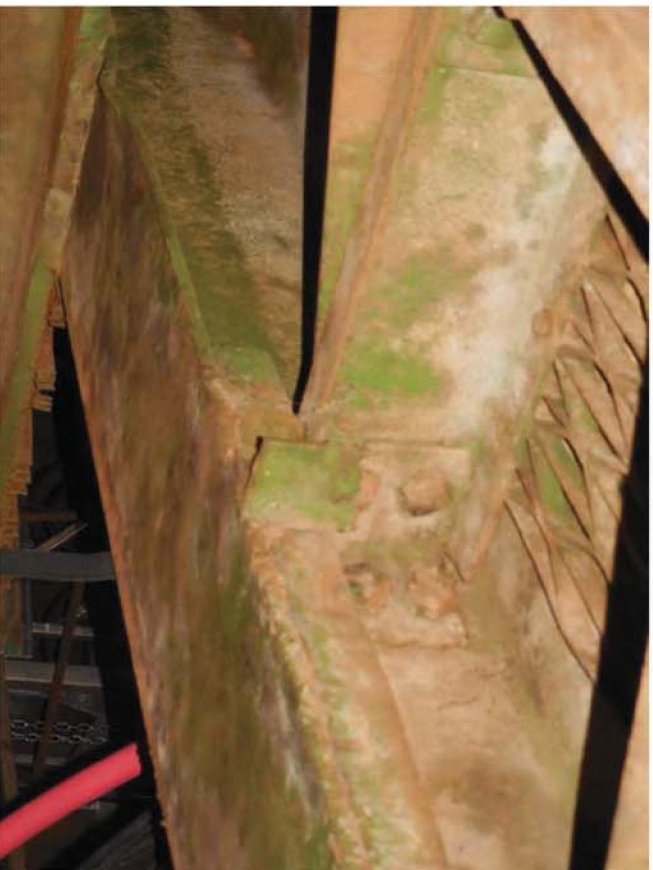
Photo 41: Tank #17 framing – Walkway framing
