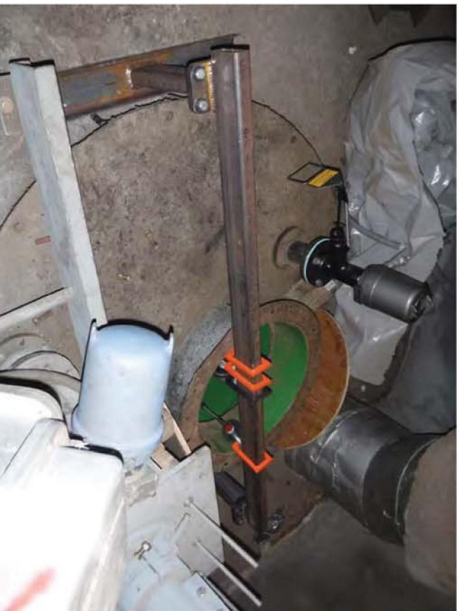
Photo 1: Spider support at top of Tank #17
