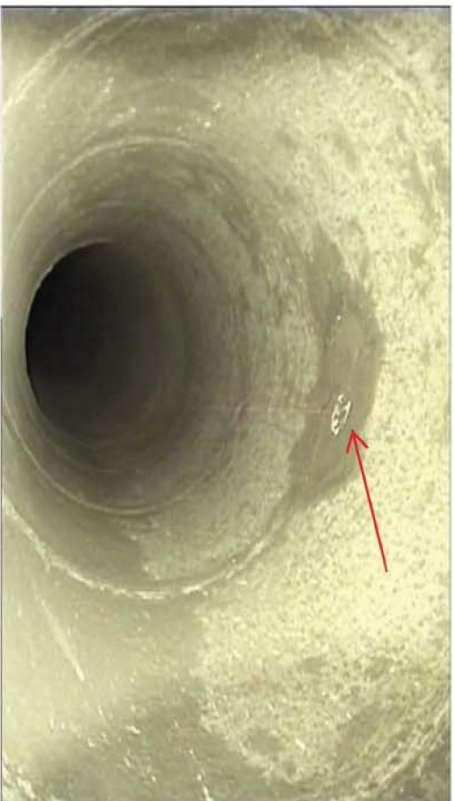
Photo 2: Large calcium deposit at top of pipe, roughly 1-2" diameter.
