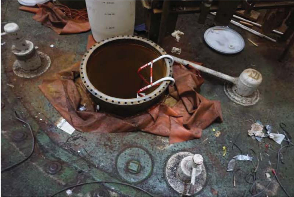
Photo 23: 32-inch piping with vortex preventer removed for inspection
