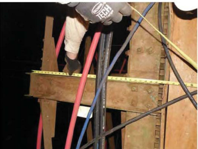
Photo 43: Tank #17 framing – Walkway framing
