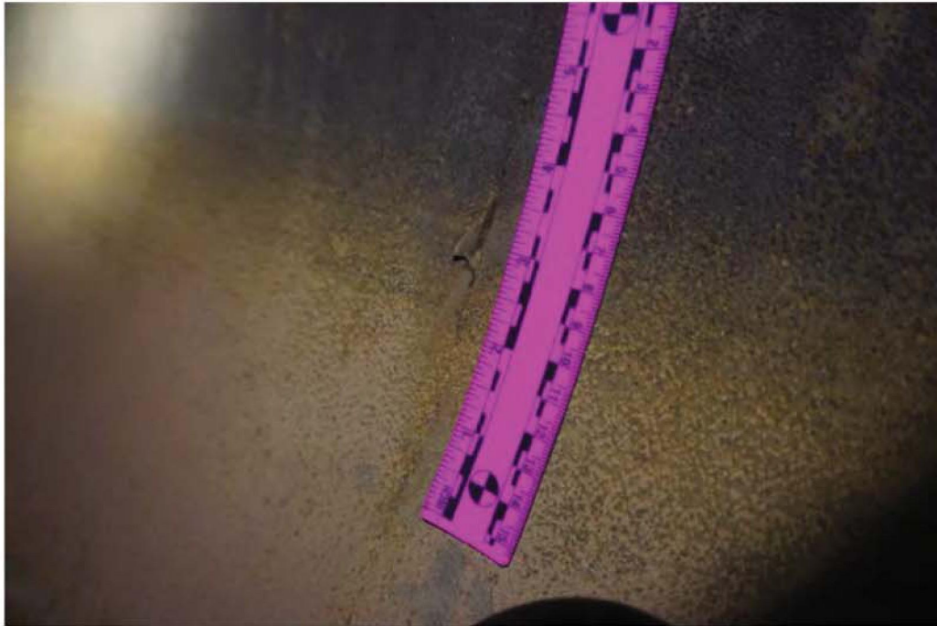
Photo 25: Weld indication in circumference weld of 32-inch line
