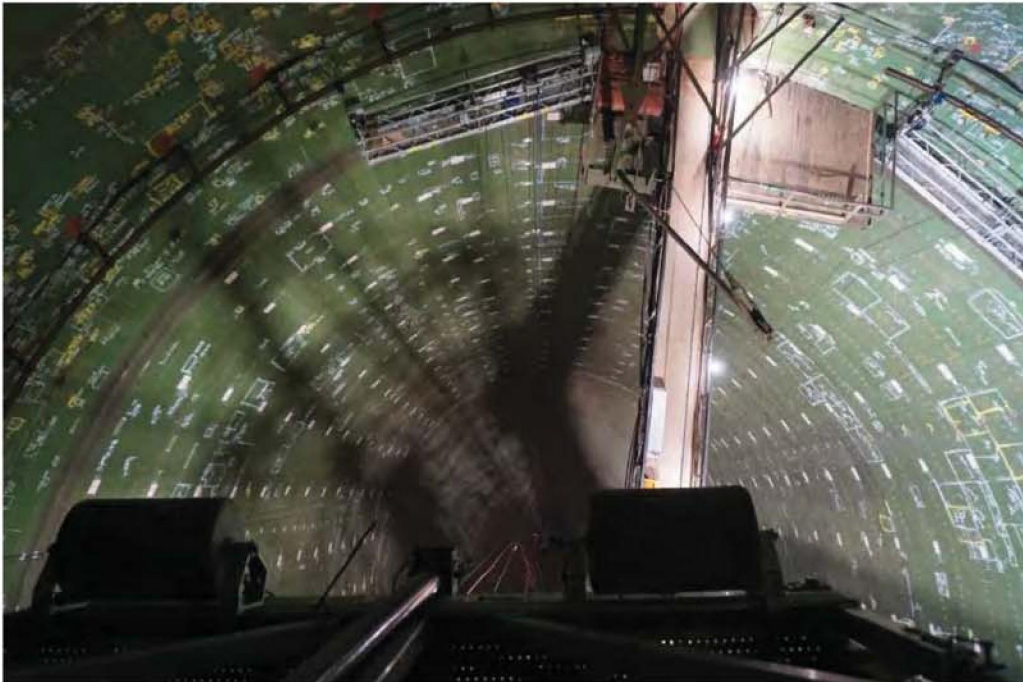
Photo 2: Catwalk to center tower
