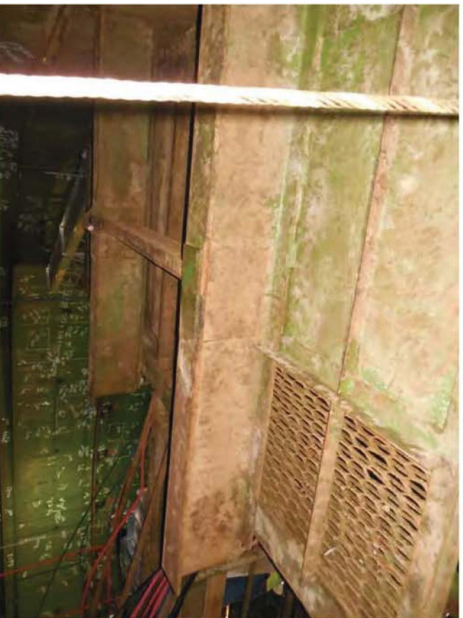
Photo 28: Tank #17 framing – entrance framing
