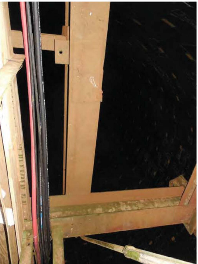
Photo 24: Tank #14 framing – entrance framing
