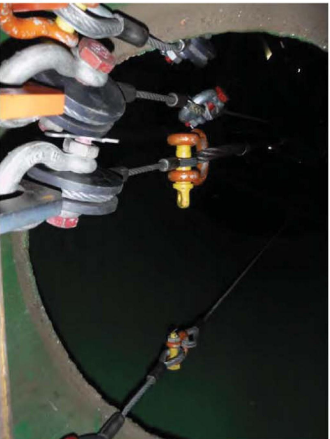
Photo 2: Tank #17 - Spider support at top
