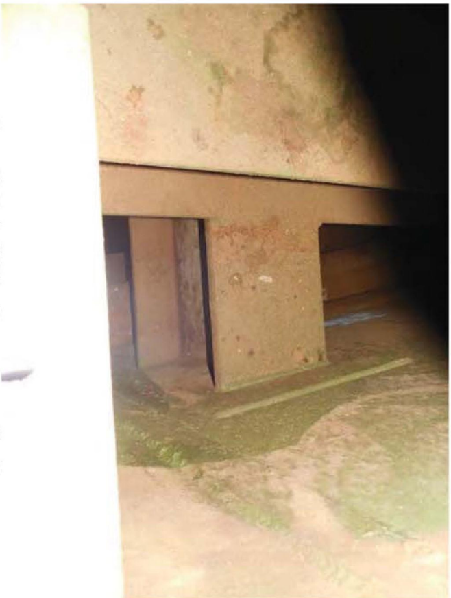
Photo 27: Tank #17 framing – entrance framing
