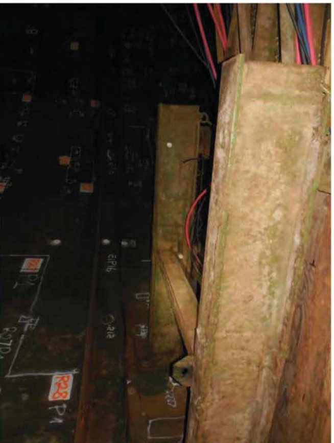
Photo 34: Tank #17 framing – entrance framing
