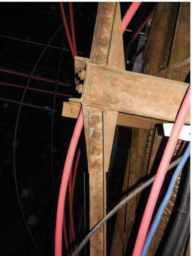
Photo 44: Tank #17 framing – Walkway framing
