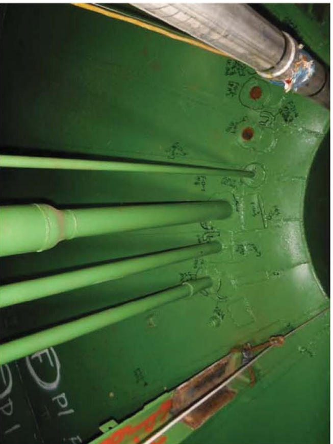
Photo 20: Tank #17 framing – tower connection to tank walls at the top
