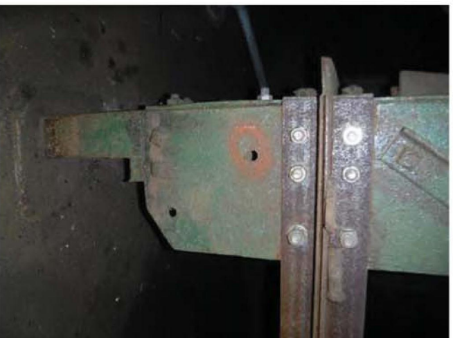
Photo 9: Tank #17 Base tower leg view
