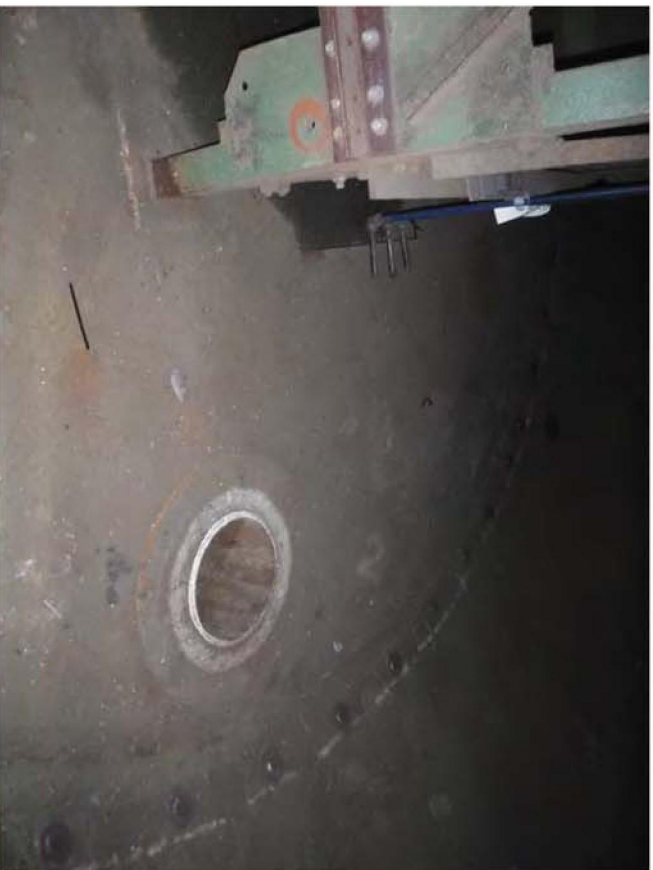
Photo 6: Tank #17 base view
