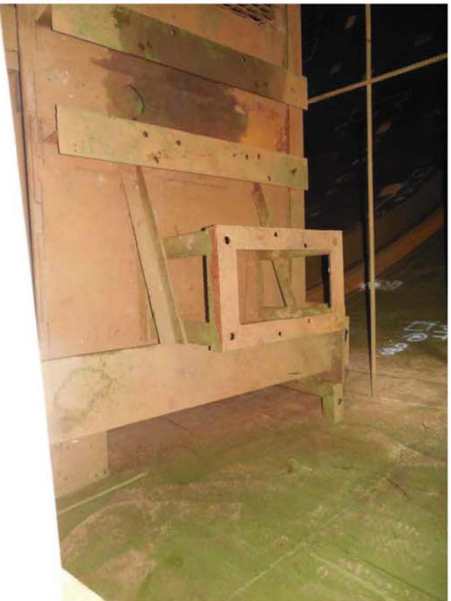
Photo 26: Tank #17 framing – entrance framing
