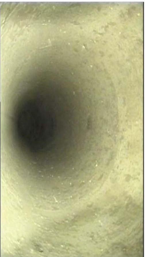
Photo 2: Large calcium deposit at top of pipe, roughly 1-2" diameter.
