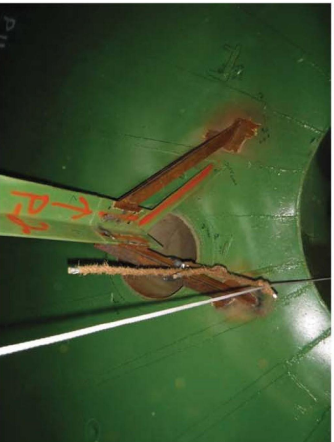
Photo 17: Tank #17 framing – tower connection to tank walls at the top
