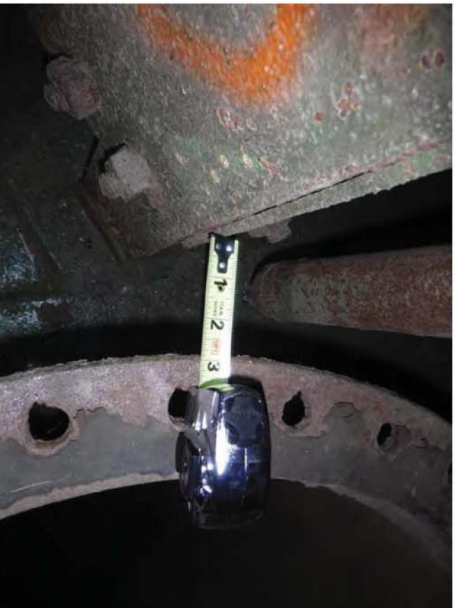
Photo 8: Tank #17 base view
