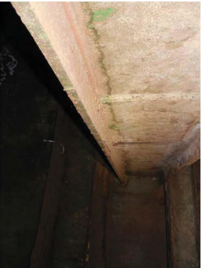
Photo 39: Tank #17 framing – entrance framing
