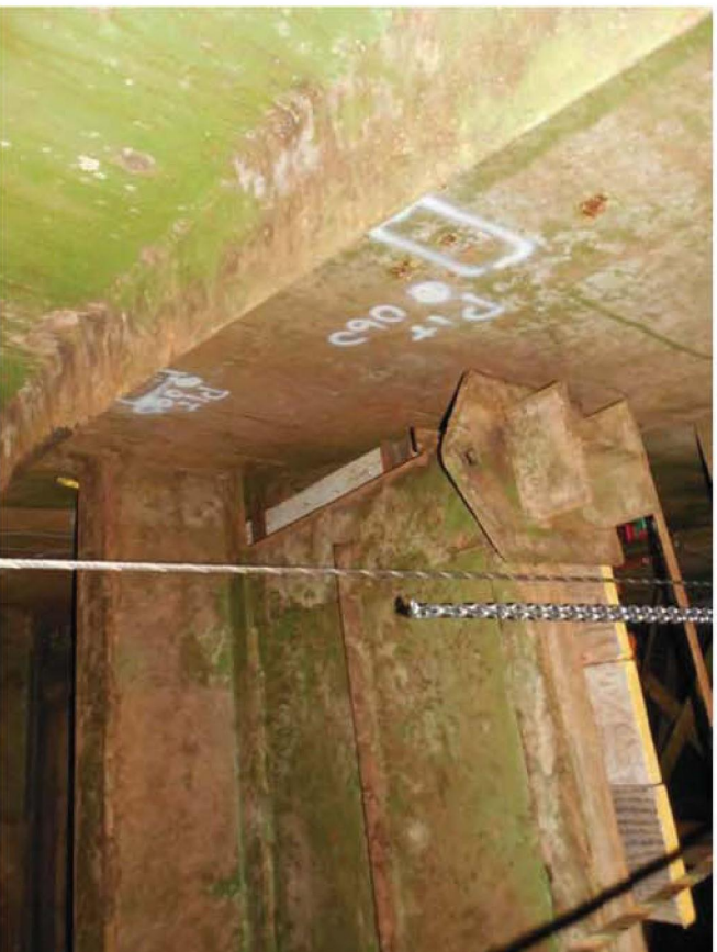
Photo 29: Tank #17 framing – entrance framing
