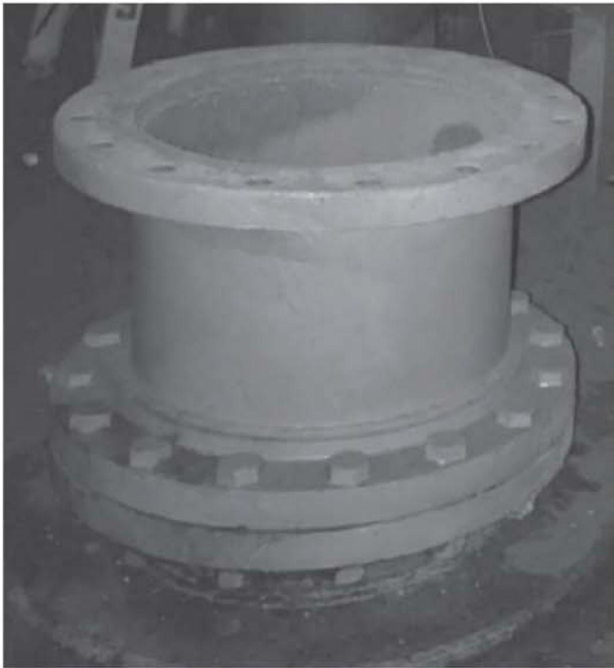
18" before blind; Blind was on top of the flanged spool for test
