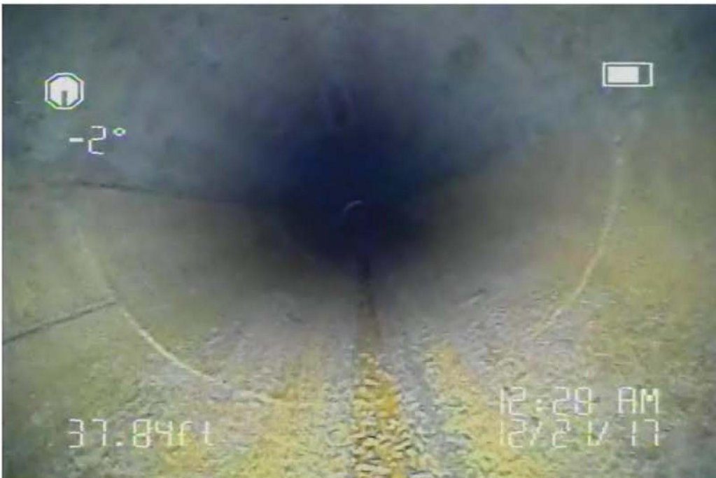
Photo 24: Visual inspection camera photo of 16-inch piping
