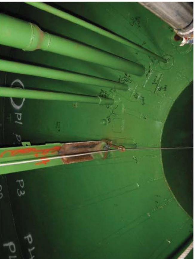
Photo 18: Tank #17 framing – tower connection to tank walls at the top
