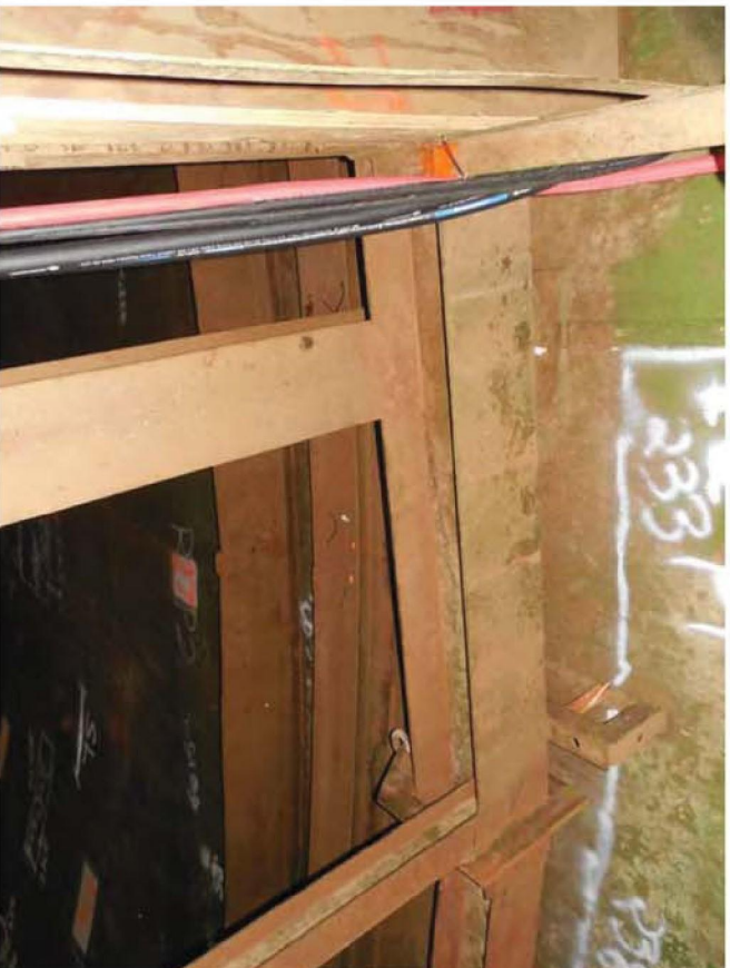
Photo 23: Tank #14 framing – entrance framing
