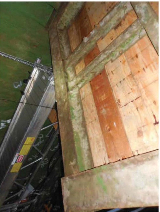
Photo 36: Tank #17 framing – entrance framing
