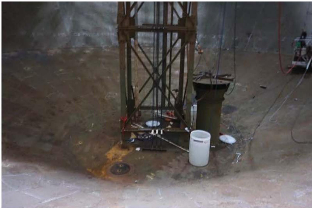
Photo 21: Tank floor and center tower
