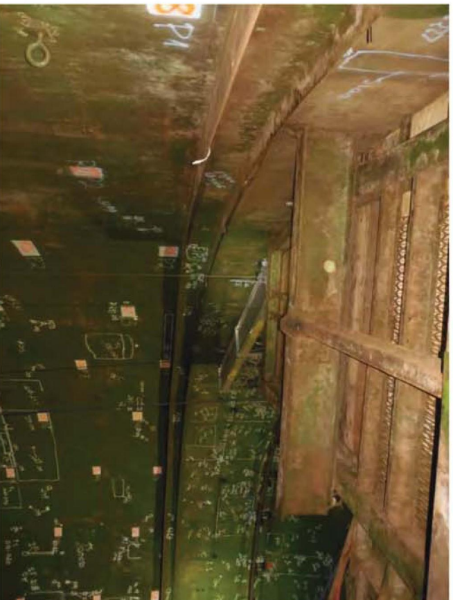
Photo 30: Tank #17 framing – entrance framing
