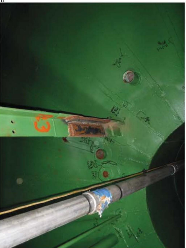
Photo 19: Tank #17 framing – tower connection to tank walls at the top
