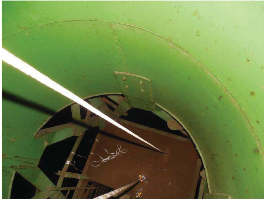
Photo 10: Tower leg connection to tank wall at the top
