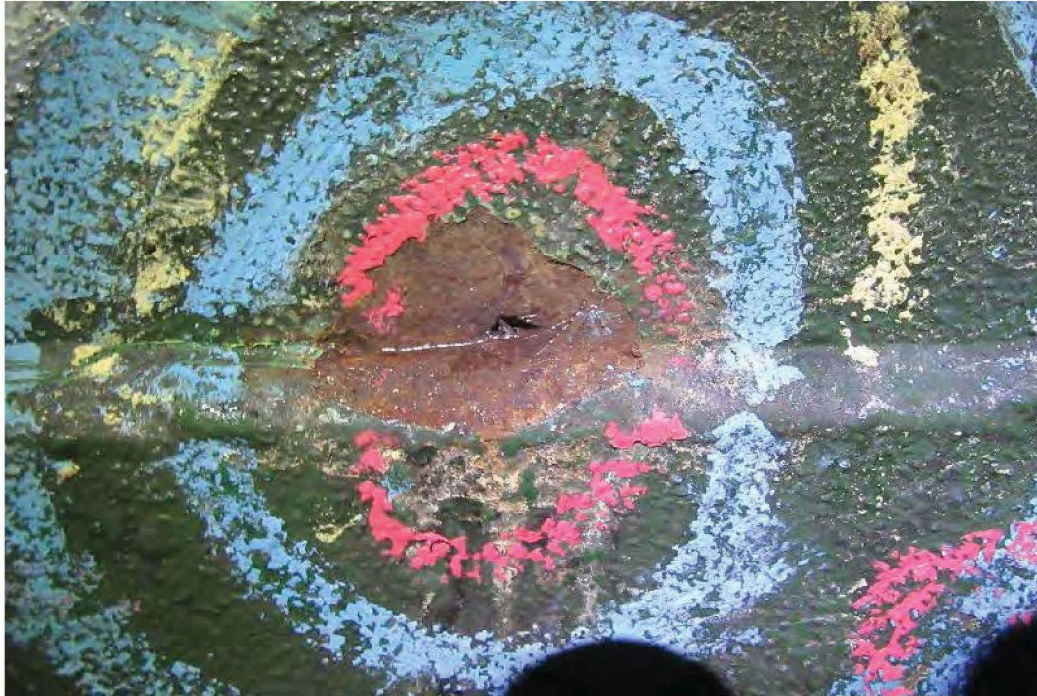
Photo 9: Liner damage in extension ring plate in course 2. The area was corroded and included coating failure at the margins. No evidence of cut marks or gouges was observed.
