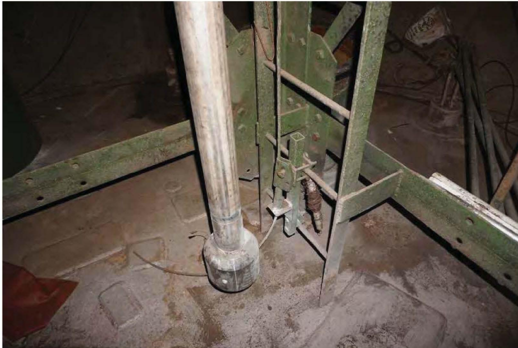
Photo 22: ATG at tank floor.
