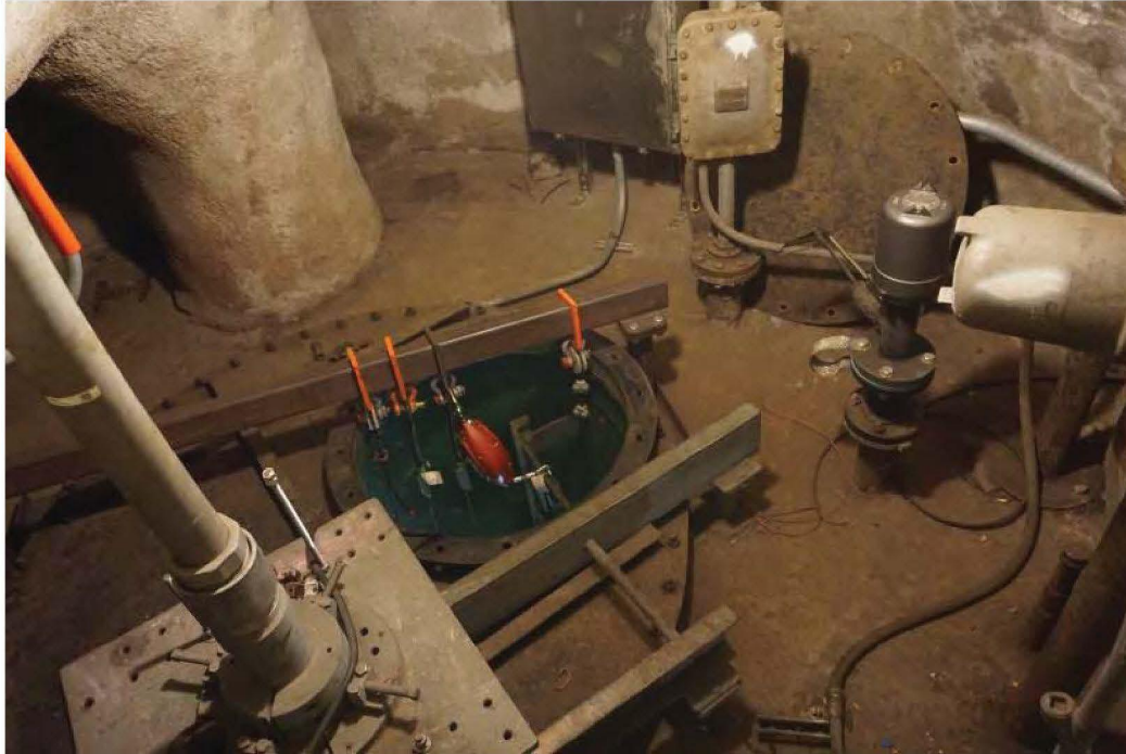
Photo 1: Upper Access Manway and tank gauges.
