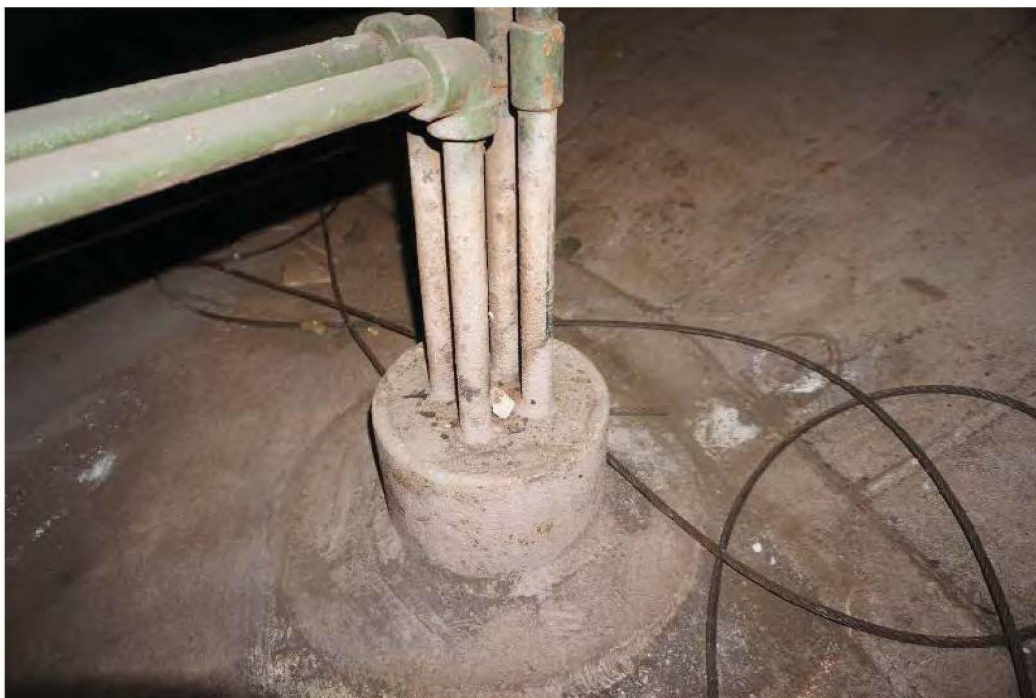
Photo 21: Sampling lines' tank floor penetration.
