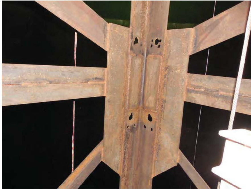
Photo 10: Multiple large holes in gusset plates at elevation 225
