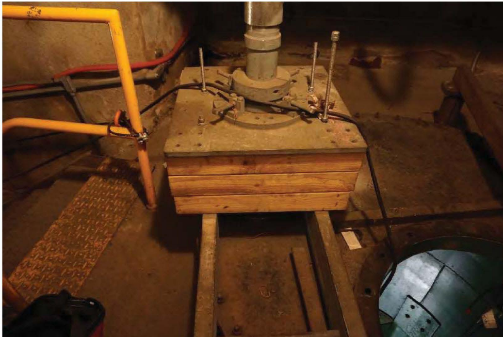
Photo 2: Cribbing supporting ATG.
