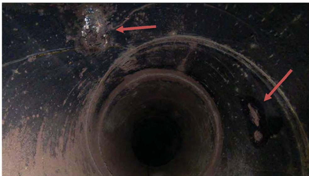
Photo 4: Several large holes on top left side of pipe with possible calcium deposit forming on closest hole.
