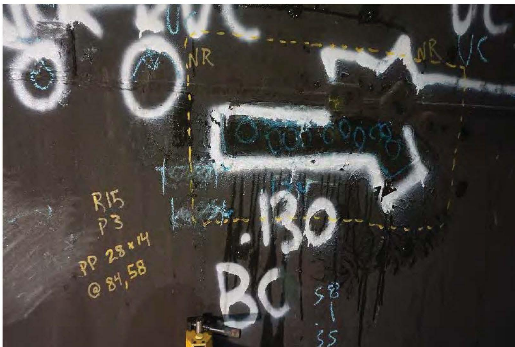
Photo 11: Layout of the extents of a patch plate (yellow dashed lines) to completely cover defects in the shell due to backside corrosion.
