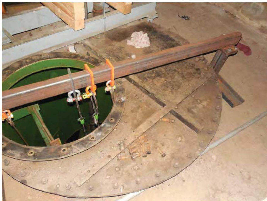
Photo 11: Support structure and cables for spider basket.
