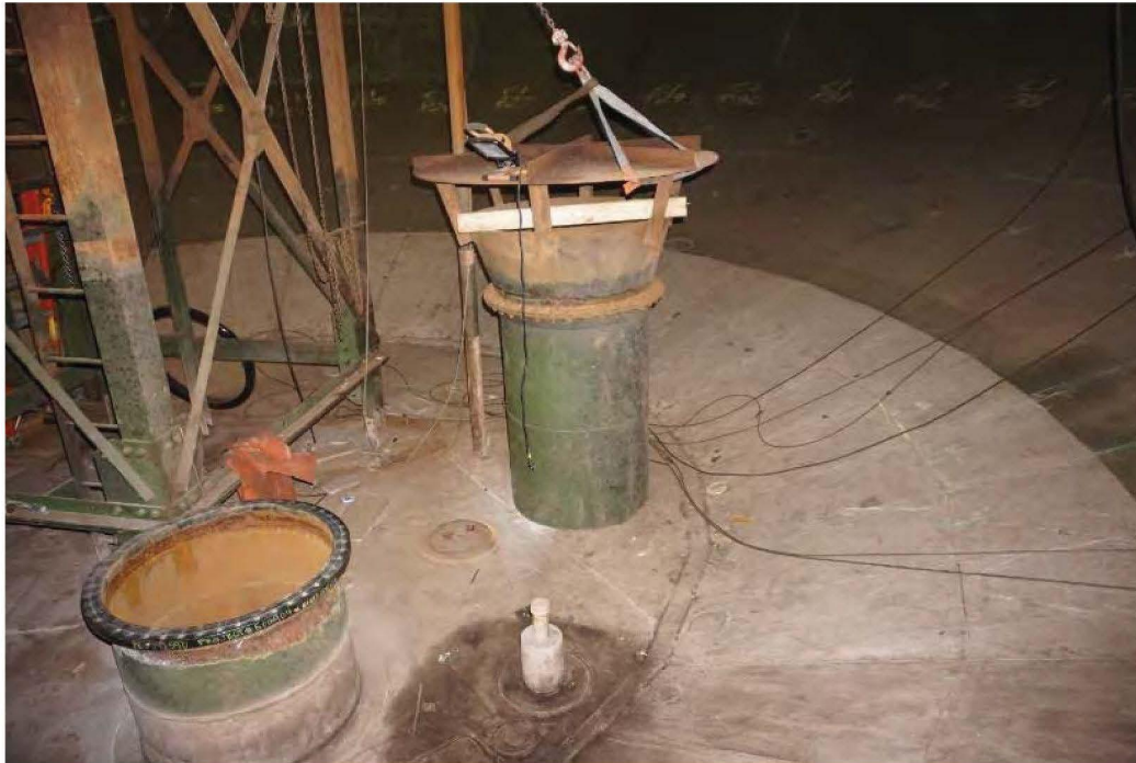
Photo 18: 32-inch piping's vortex preventer removed.
