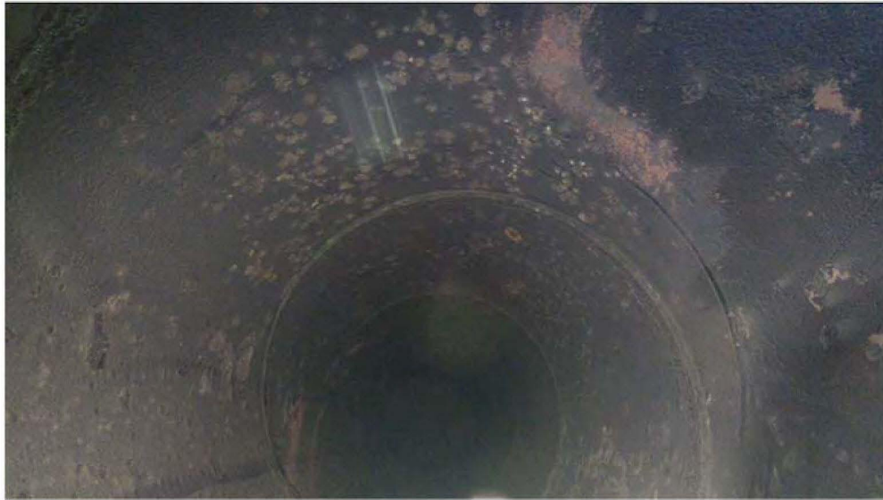
Photo 2: Widespread pitting throughout ventilation line.
