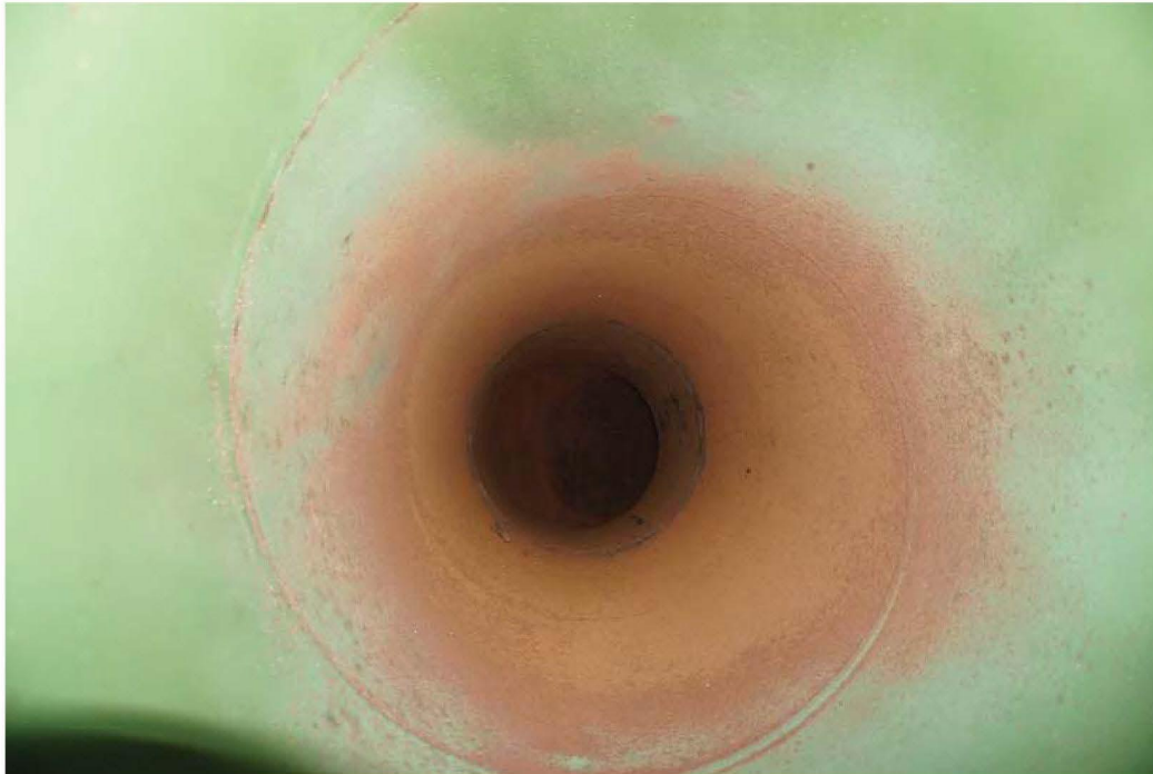
Photo 3: Vent piping from upper dome near upper access manway.
