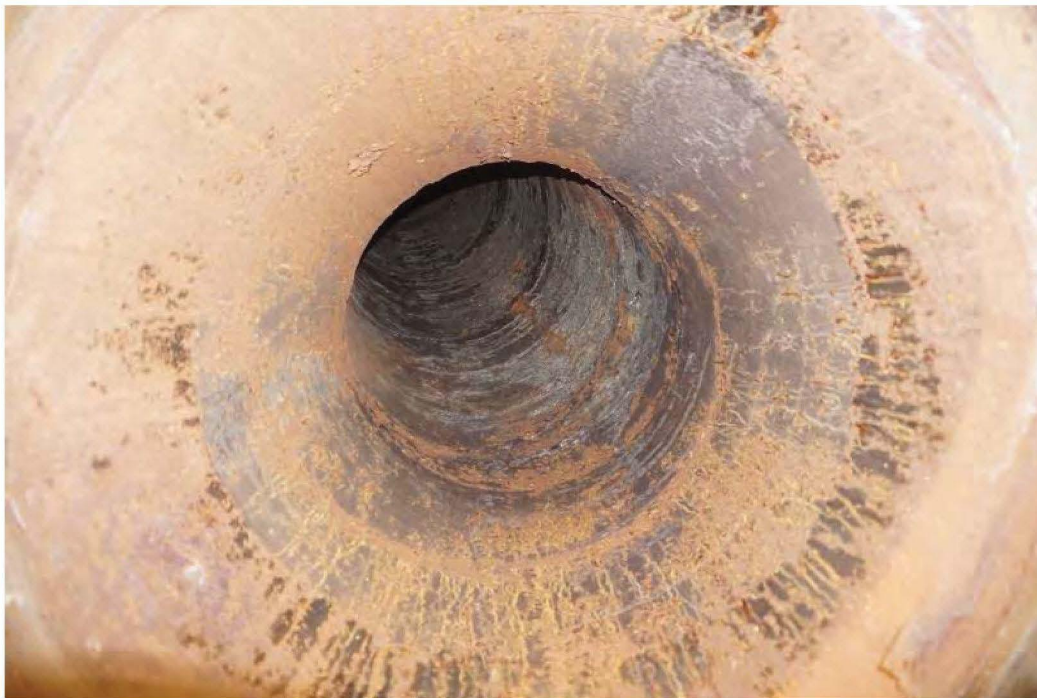
Photo 6: Internal condition of vent piping as seen from upper access tunnel.
