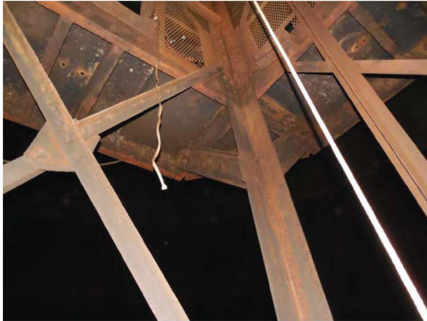
Photo 6: Underside view of walkway framing
