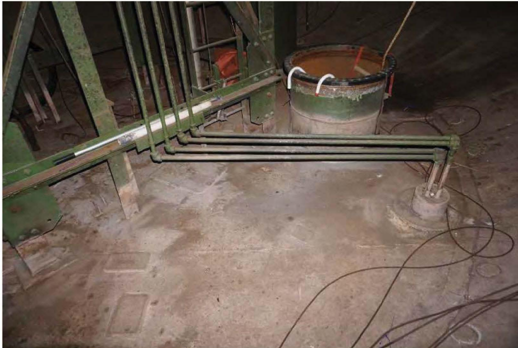
Photo 20: Sampling lines at tank floor.
