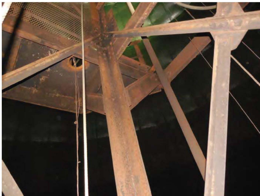
Photo 7: Underside view of walkway framing
