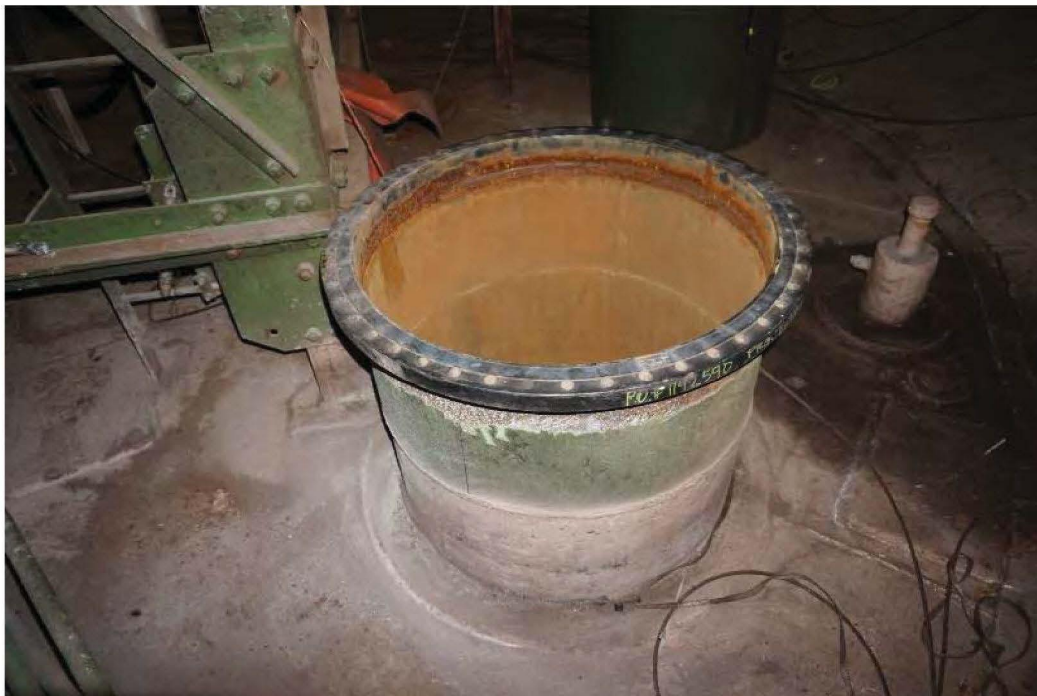
Photo 17: 32-inch piping at tank floor with vortex preventer removed with new flange installed.
