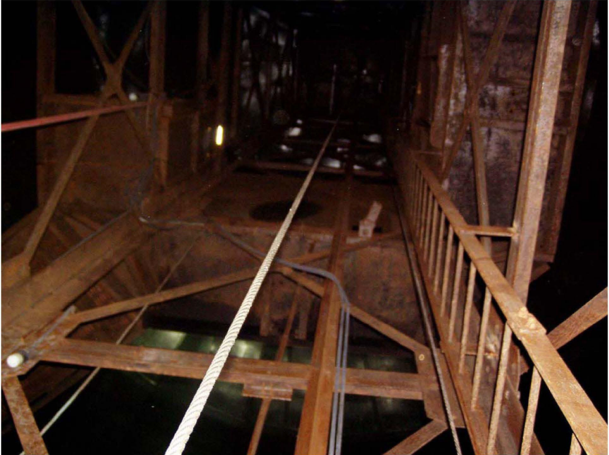
Tank 15 relocated ladder – note the clips attaching the ladder to the tower.
