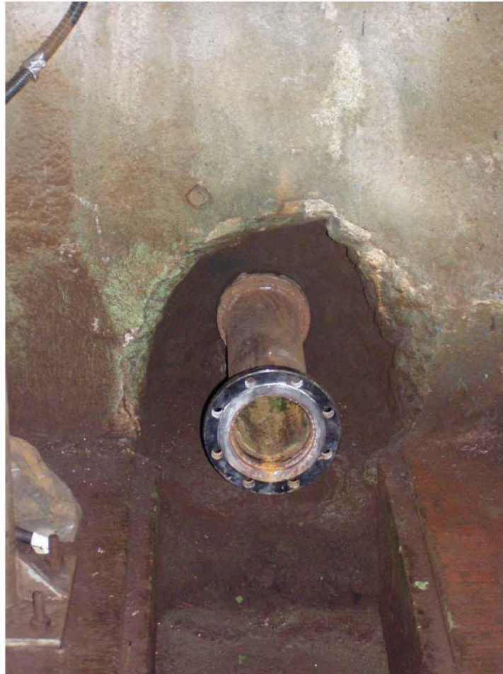
View of new slop line from lower tunnel before installation of 6" valve.
