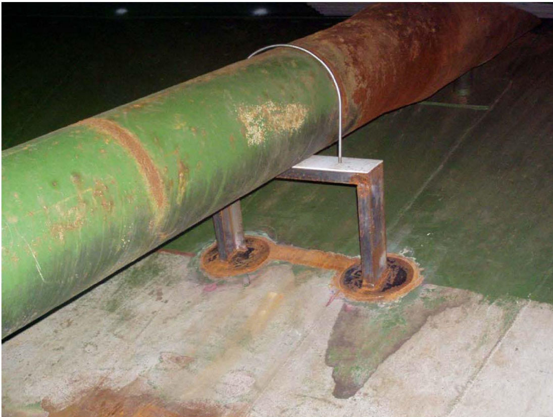
New 18" line support with re-pads
