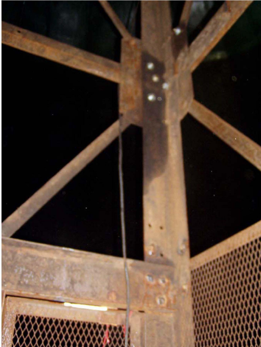
Typical area of replaced fasteners - note plug weld repair of flame cut holes.
