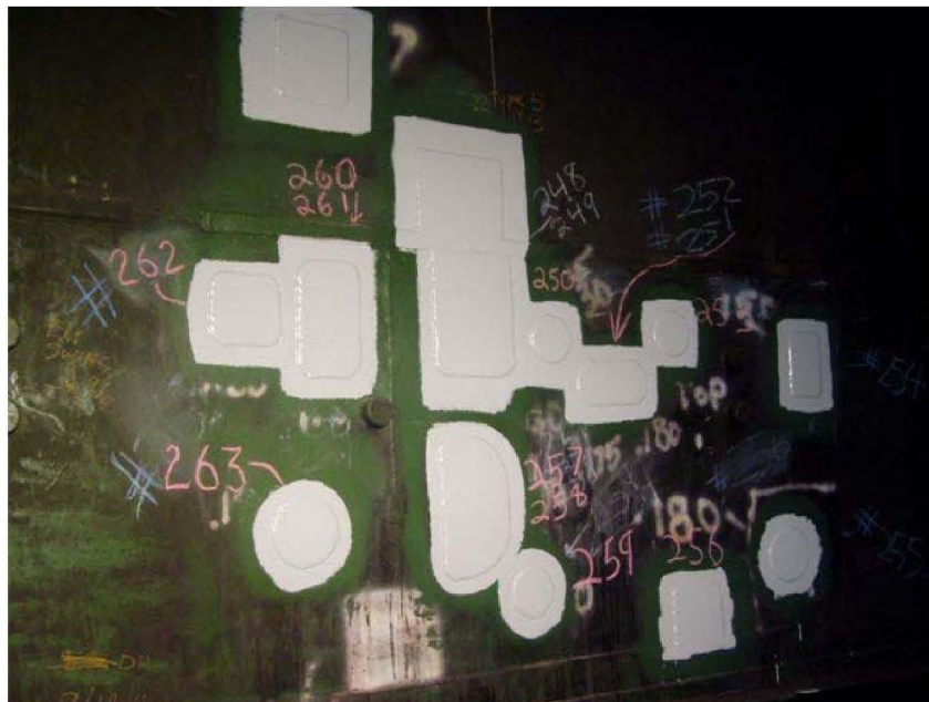
Typical patch plate repairs (note the Dunkin & Bush assigned flaw numbers)
