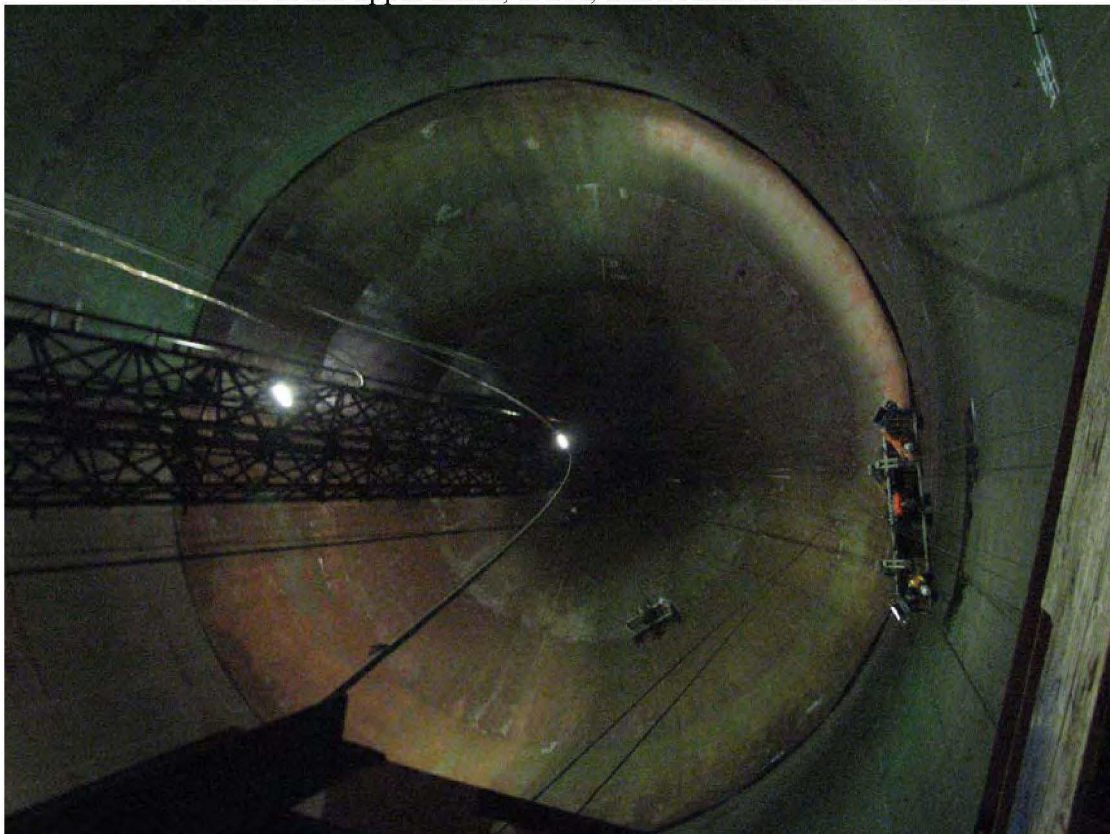
Looking down at the lower dome and the crew inspecting under the catwalk.
