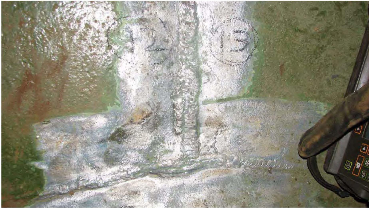
Intersecting welds between plates 12 and 13 of course 1 and the floor.
