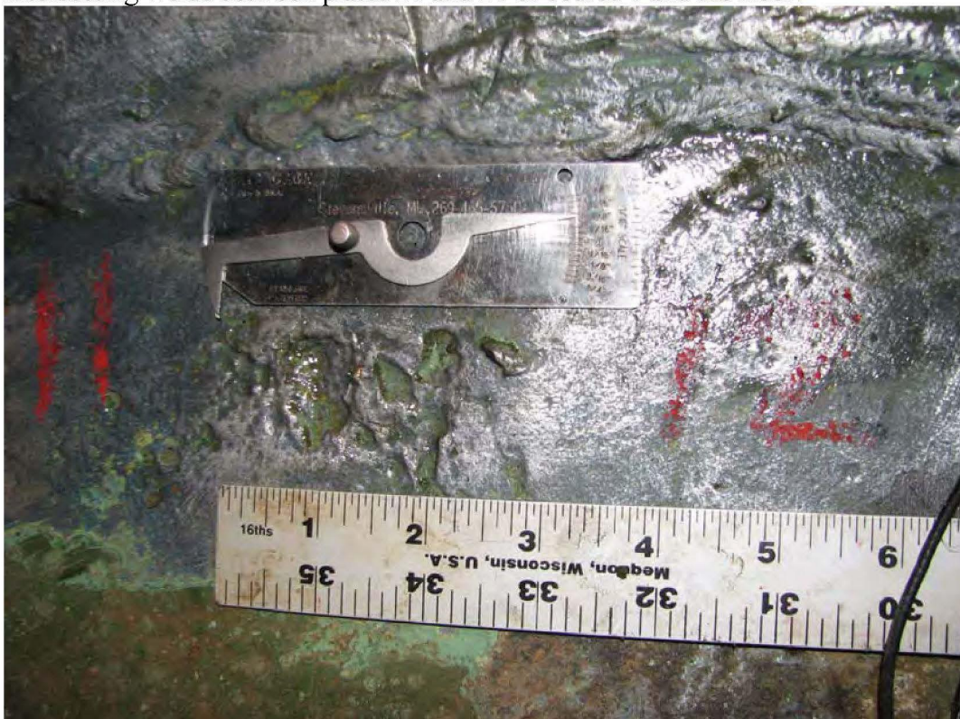
Flaw # 83, topside pitting on plate 4 of the floor, 0.336" remaining, near plates 11 and 12 of course 1
