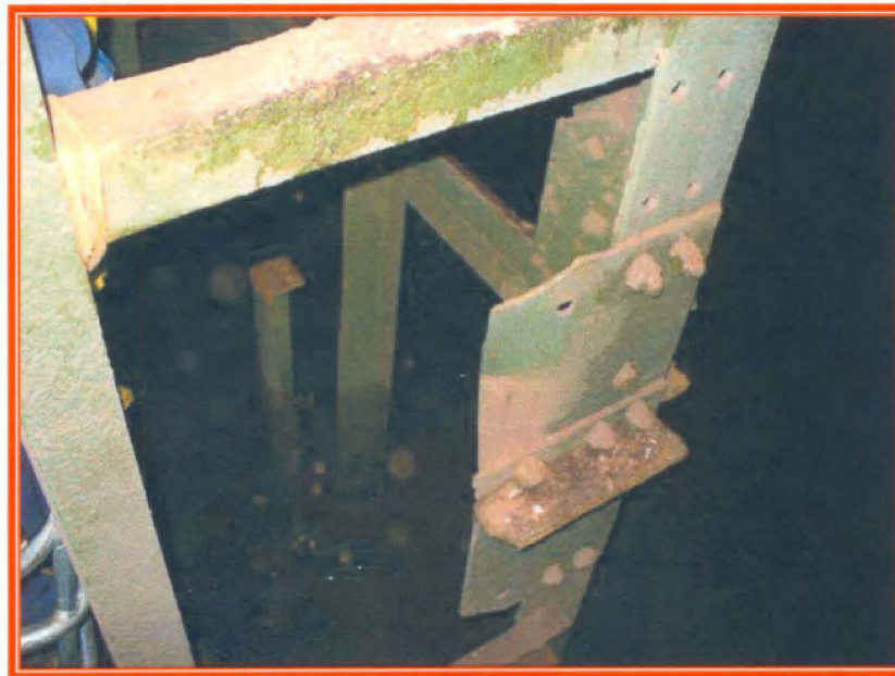
Photo #8: Missing diagonal
