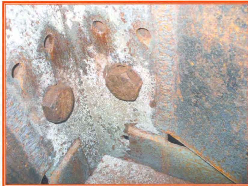
Photo #2: Visible slippage of the bolt connection
