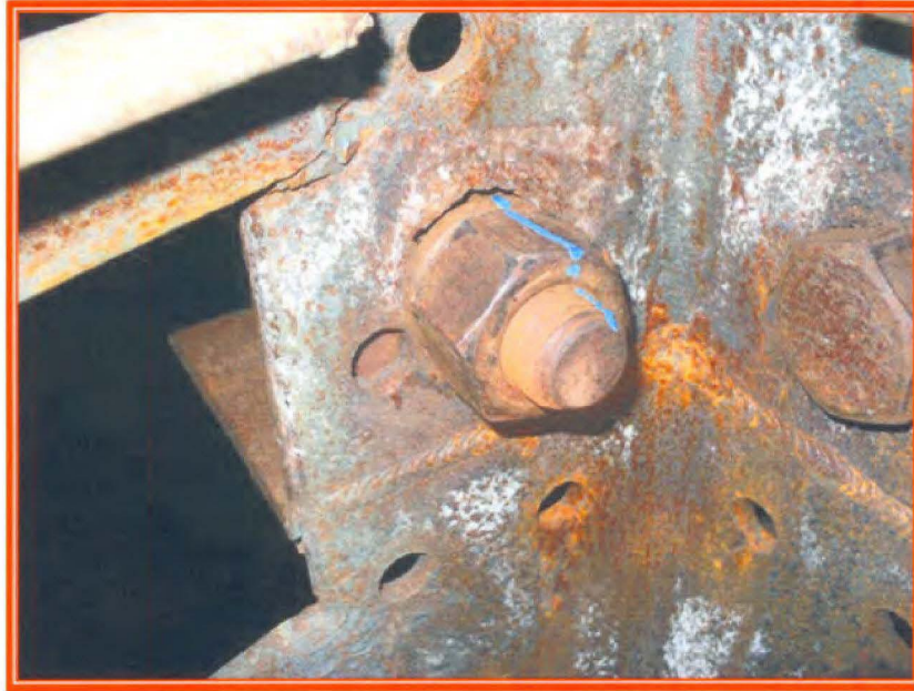
Photo #1: Visible slippage of the bolt connection
