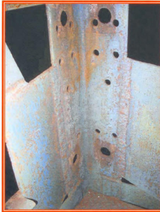
Photo #3: Big holes on the framing members
