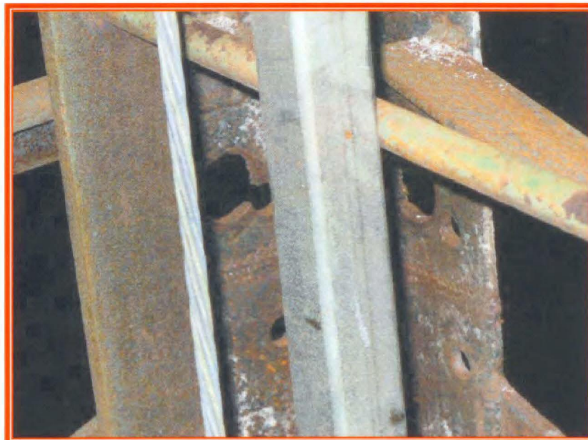
Photo #4: Big holes on the framing members
