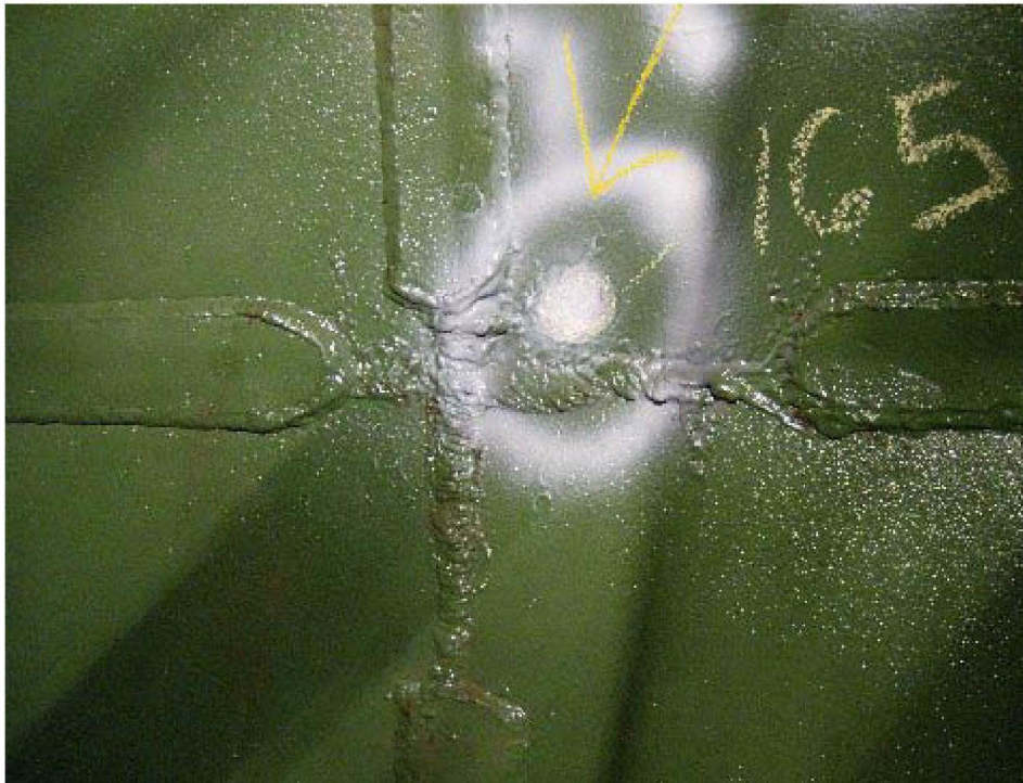
Flaw 304 Loss of Wall measured .165"
