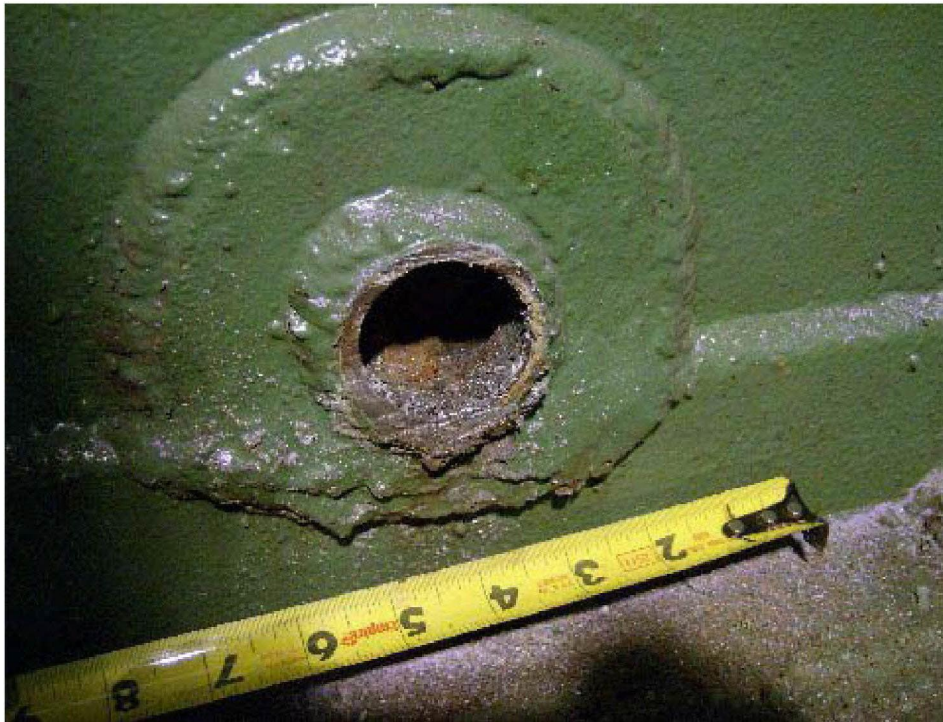
One of approximately Six Hundred piping penetrations that were removed requiring repair
