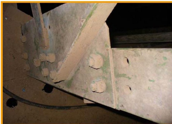
Image 1: Showing Tank #20 Tower frame and boom missing members and bolts
