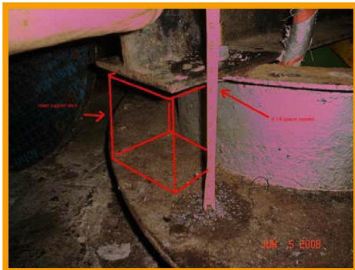
Image# 5: Showing Tank #20 Top Anchor I-Beam shortened and supported.
