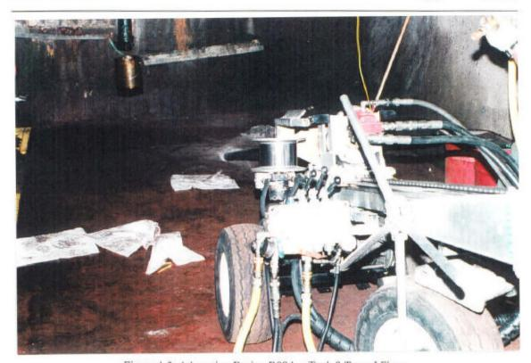
Figure 4-3 Advancing Boring B09A - Tank 9 Tunnel Floor
