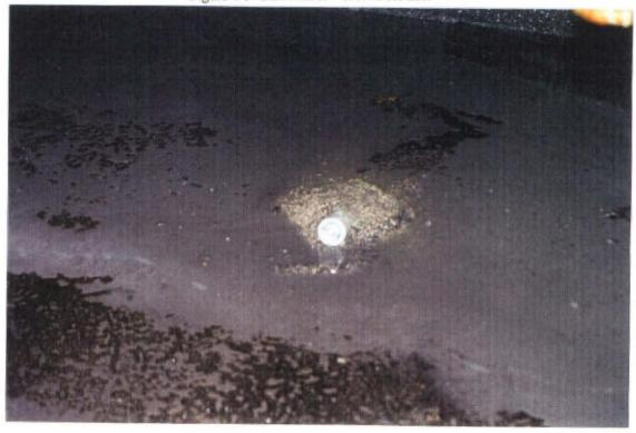
Figure 4-6 Typical Completed Boring with PVC CAP 4-10
