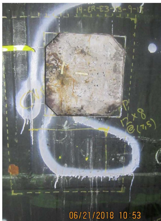
Figure 4-8 Location of Coupon 3 after Removal
