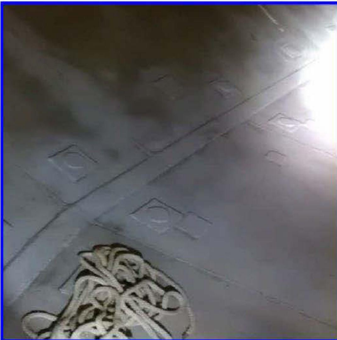
Overview of welded 4\"X4\" welded plate on lower course IR-1
