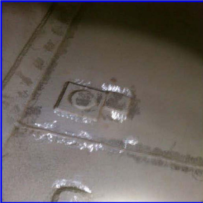
Welds and 4"X4" plate that had the weld spatter grinded off
