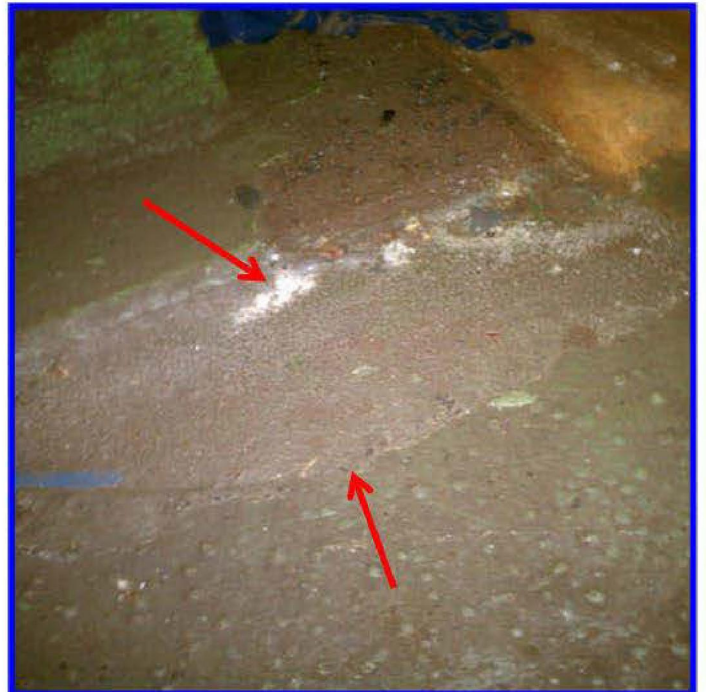
Visible salt on flat bottom of tank
