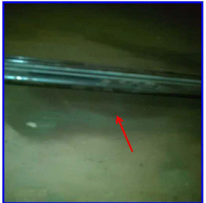
Visible grease under newly installed ppg CSI Coating Inspection Report Page 4
