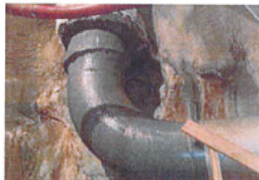
Ventilation System – Area repaired where foam was installed for ducting. Metal sheeting installed and sealed for ventilation process.
