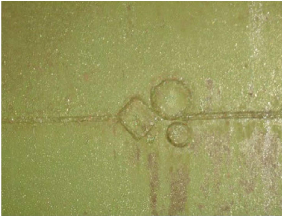
Existing Lap Patches in the Barrel section of tank 20 Note: Coating condition
