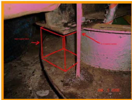
Image# 5: Showing Tank #20 Top Anchor I-Beam shortened and supported.
