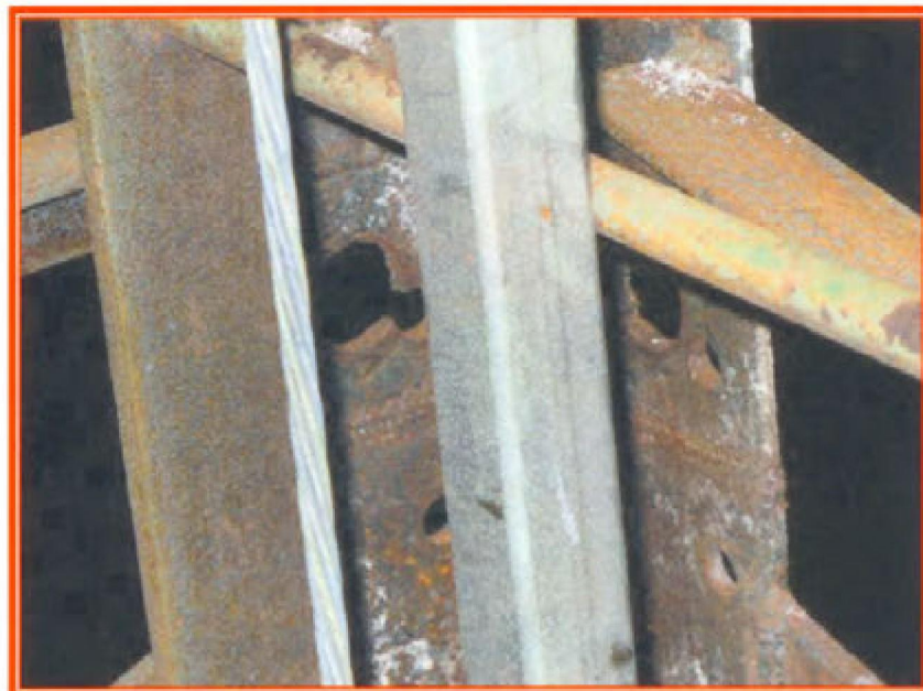
Photo #4: Big holes on the framing members
