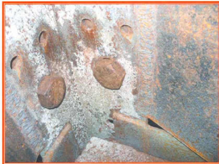
Photo #2: Visible slippage of the bolt connection
