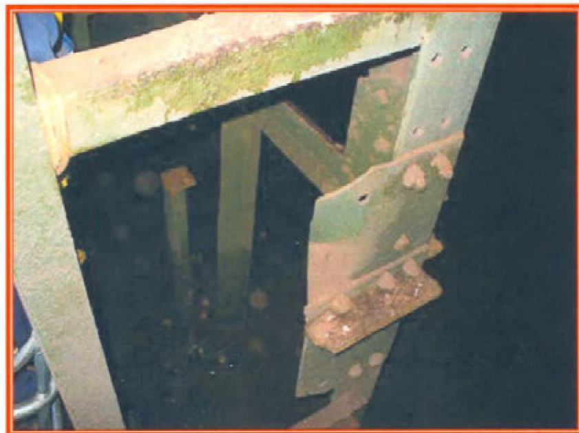
Photo #8: Missing diagonal
