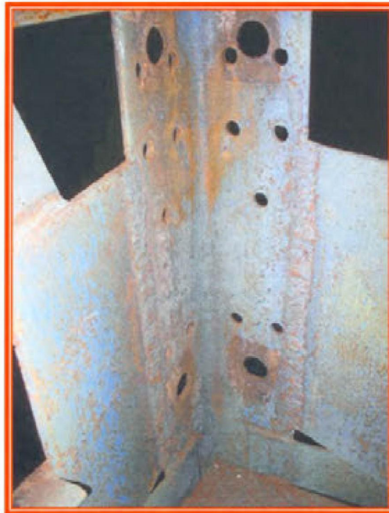
Photo #3: Big holes on the framing members
