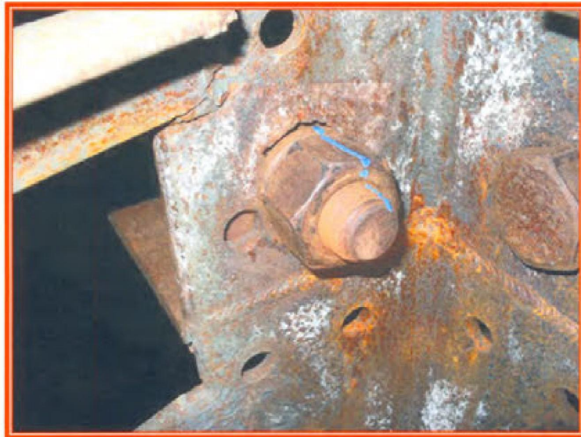
Photo #1: Visible slippage of the bolt connection
