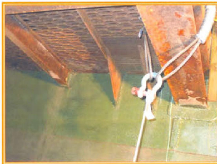
Photo #3: Weld of the major I-beam is in good condition
