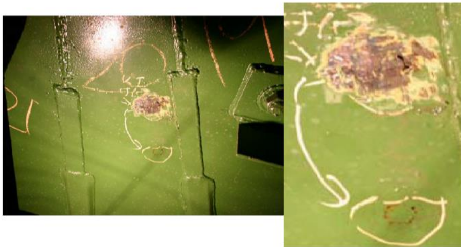
Figure 5. Photographs extracted from the API Tank 16 Inspection Report (Photograph 8) showing "holes at the top of course F of the upper dome".
