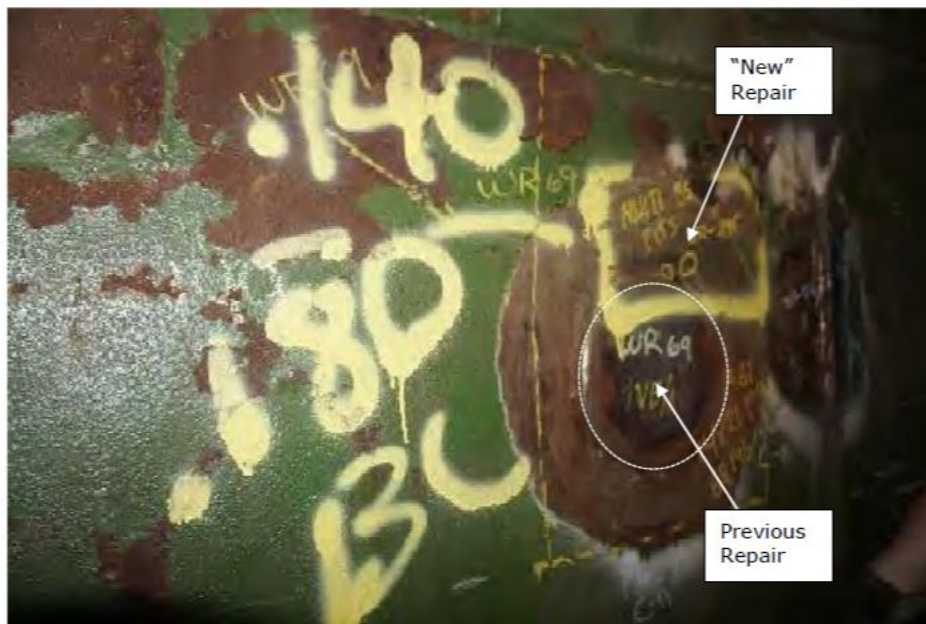
Photo 29: Backside Corrosion around existing patch plates
