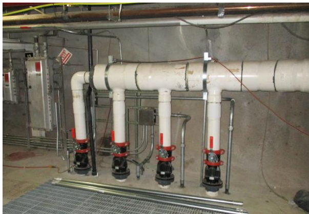
Original AFFF Retention Line Piping in Immediate Area of an AFFF Sump
