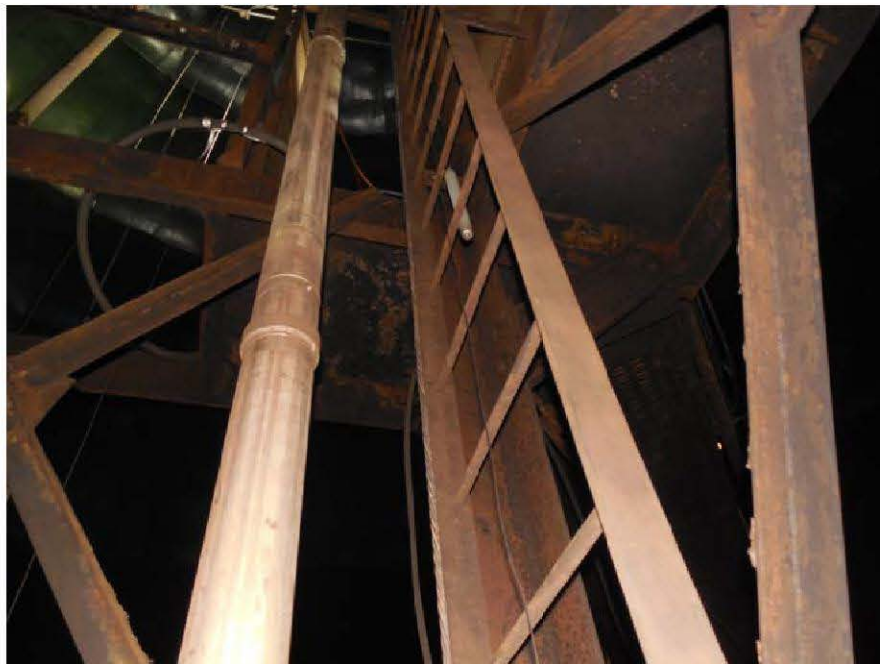
Photo 8: Underside view of walkway framing
