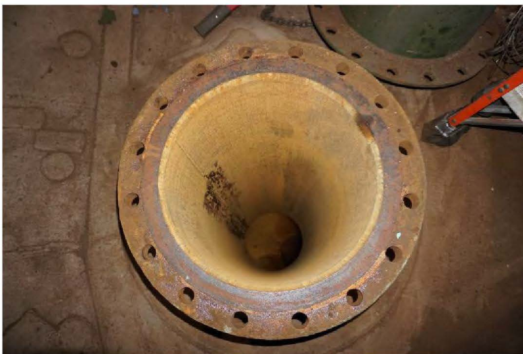
Photo 15: 18-inch piping at tank floor with diffuser removed.
