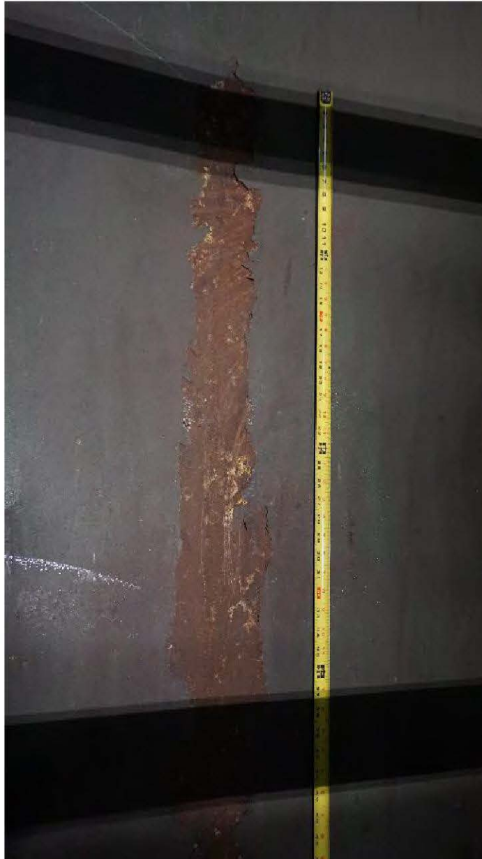
Photo 13: Large coating failures along lower dome. Re-coating to be addressed as part of the SOW.
