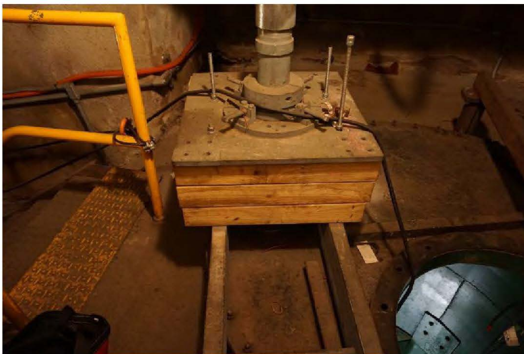
Photo 2: Cribbing supporting ATG.
