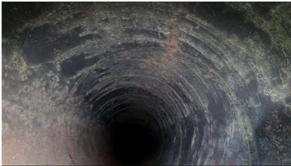
Photo 1: General corrosion and scaling of the top of ventilation line.
