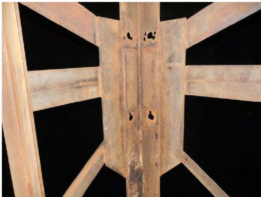
Photo 11: Multiple large holes in gusset plates at elevation 225
