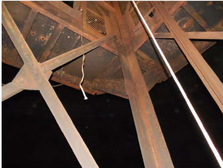
Photo 6: Underside view of walkway framing
