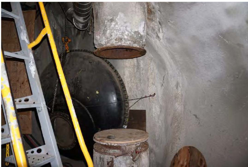
Photo 4: Vent piping with spool removed in upper access tunnel.
