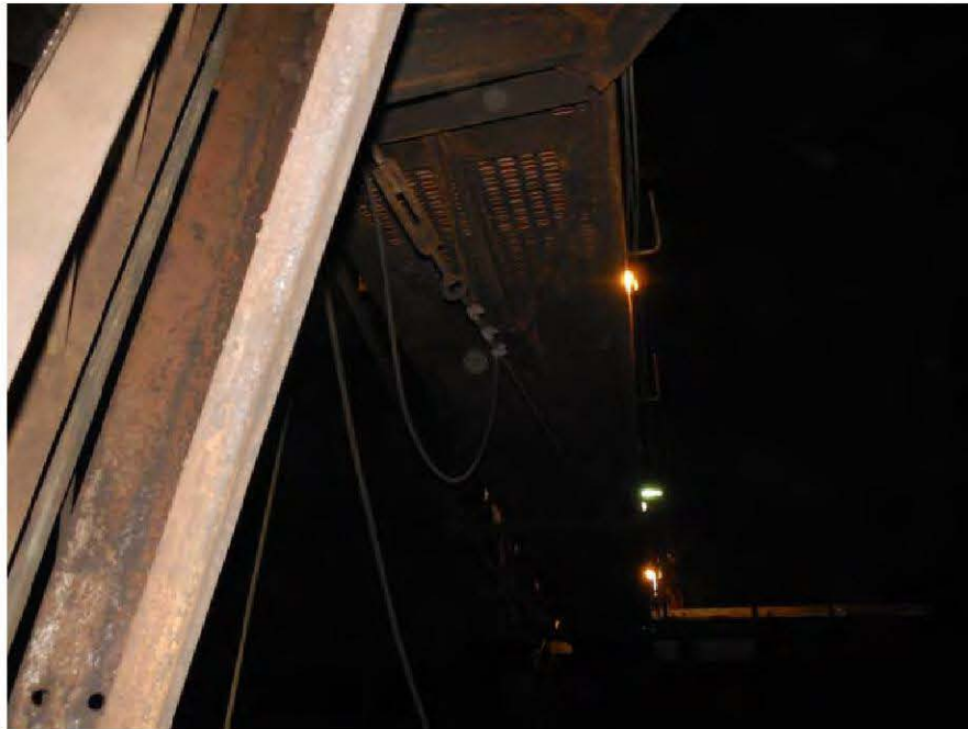
Photo 10: Underside view of walkway framing
