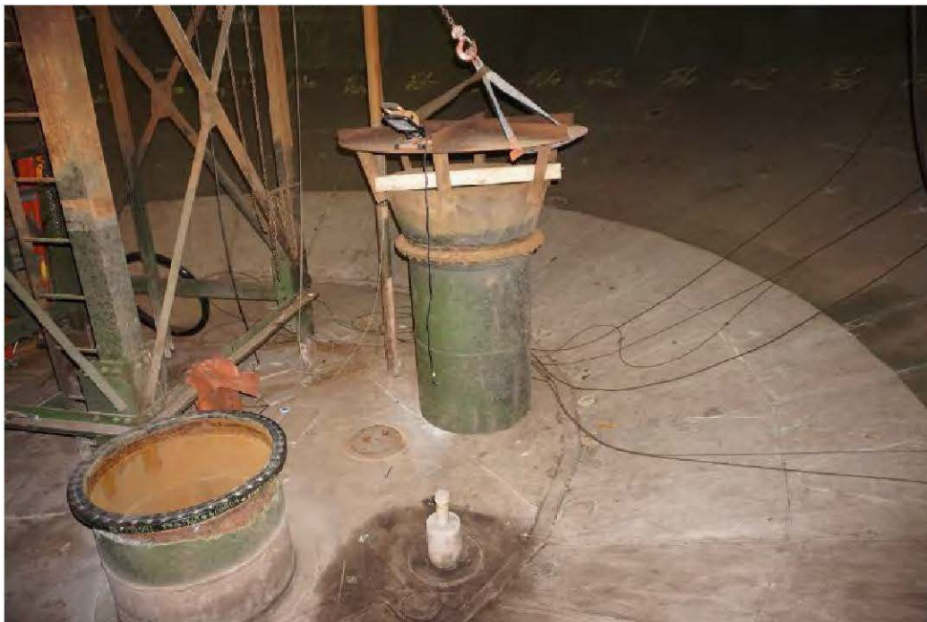
Photo 18: 32-inch piping's vortex preventer removed.
