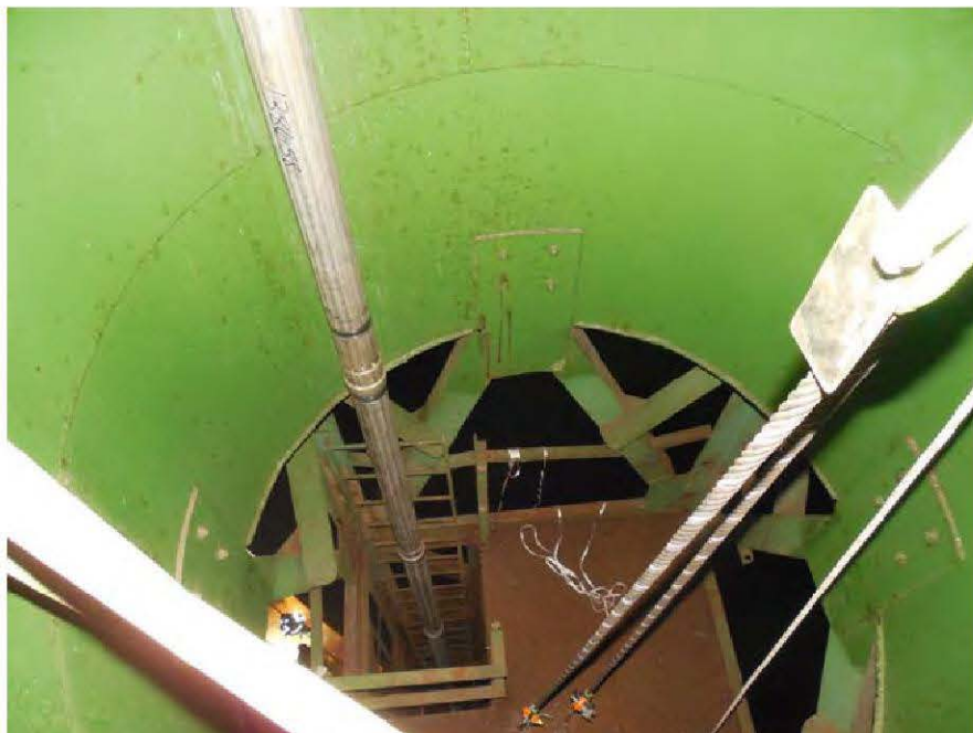
Photo 11: Tower leg connection to tank wall at the top
