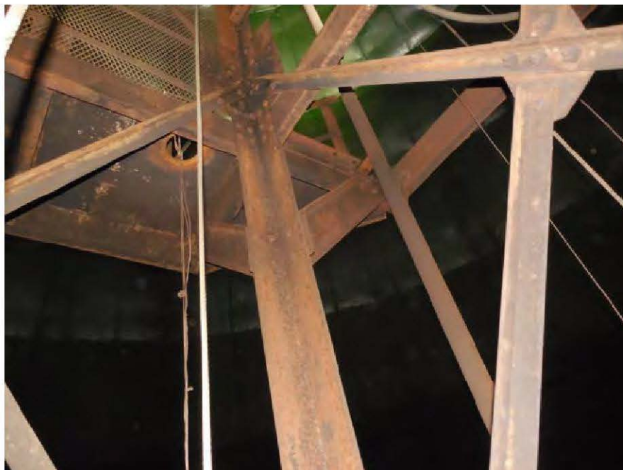
Photo 7: Underside view of walkway framing
