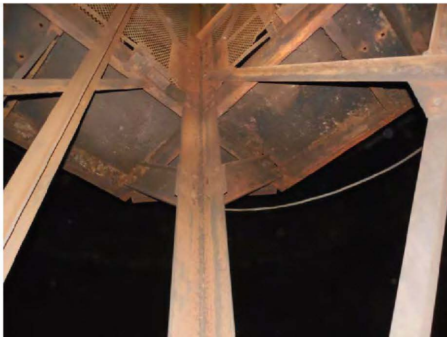
Photo 5: Underside view of walkway framing
