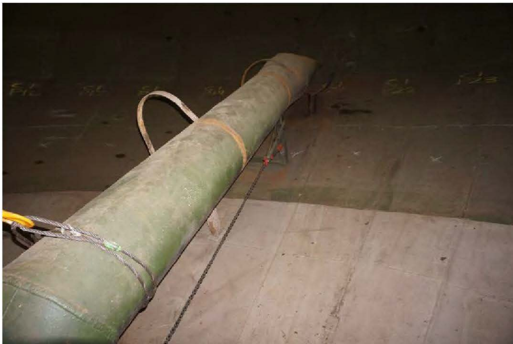
Photo 16: 18-inch piping's diffuser removed to inspect pipe supports.
