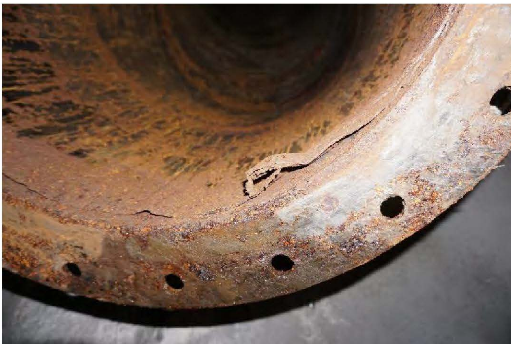
Photo 5: Flange of vent piping.
