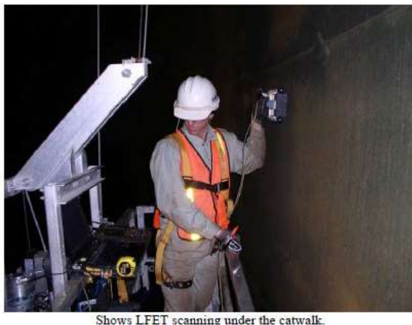
Figure 2. Photograph showing the application of the hand-held scanner used to perform LFET [B-190].
