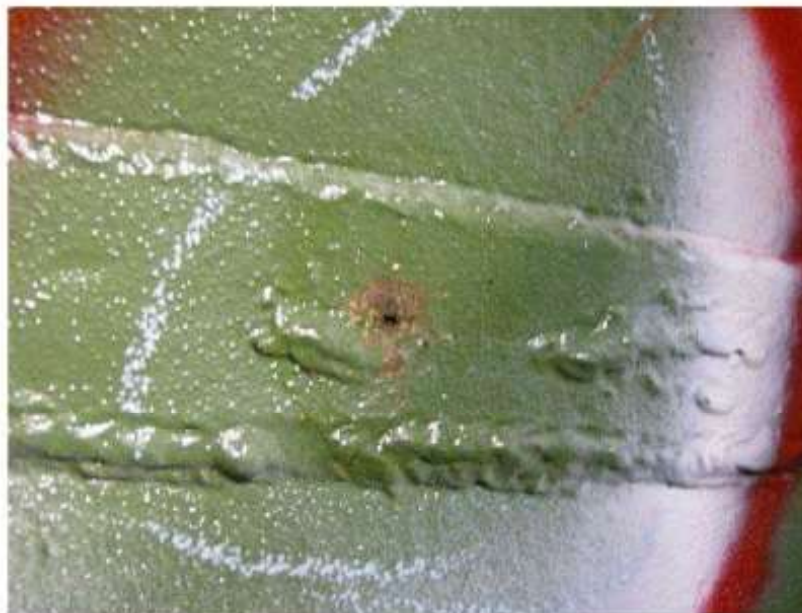
Flaw 347 through hole in strap
