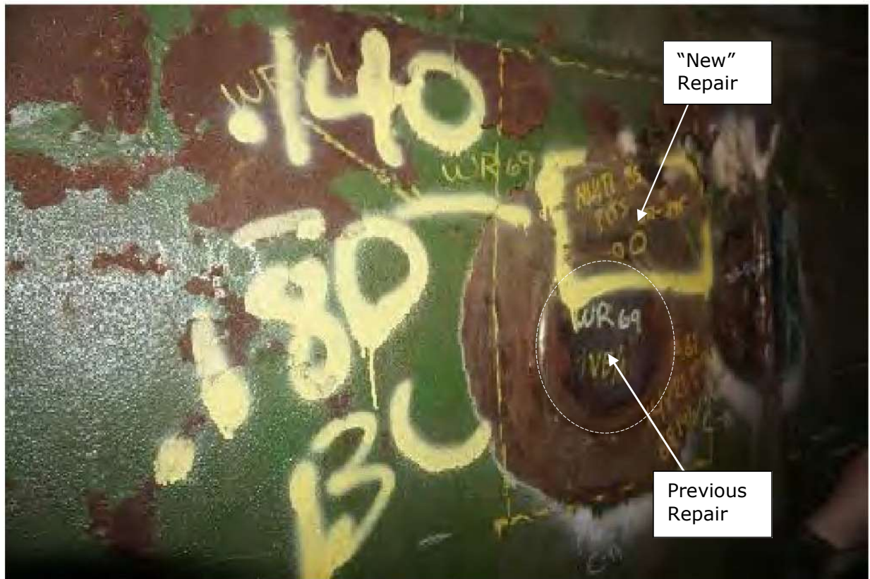
Photo 29: Backside Corrosion around existing patch plates
