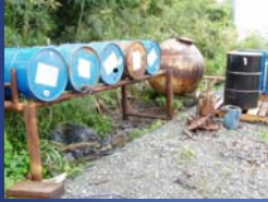
Bad No Secondary Containment No Overhead Cover
