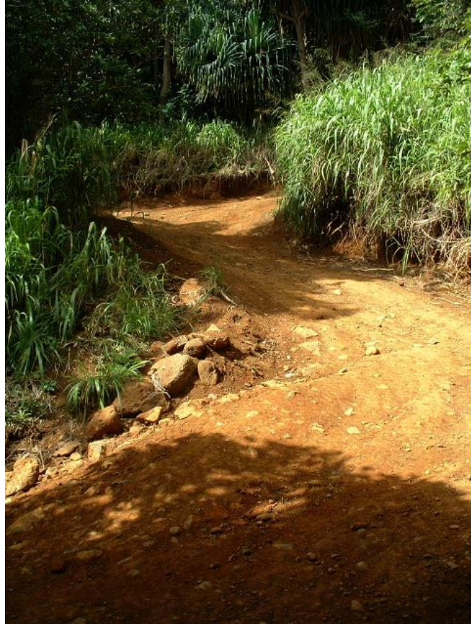
Figure 11. A steep part of a road for an ATV. Water runoff occurs in the bottom left corner of the picture. Erosion can be also seen in the same corner.
