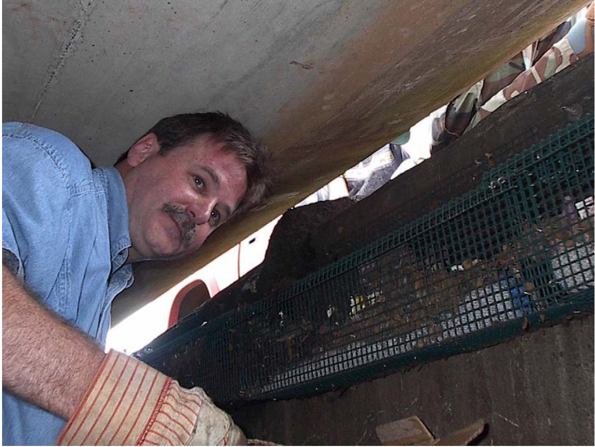
Figure 12. Paul Geisert of the the Nawiliwili Bay Watershed Council maintaining catch basin insert on Kuhio Highway
