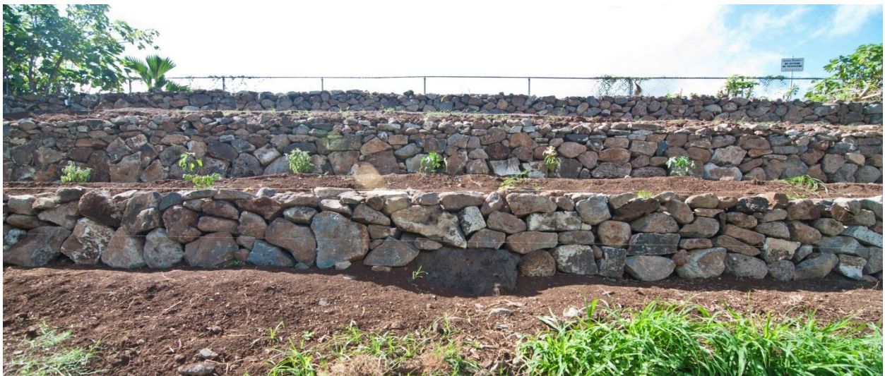
Figure 5: Traditional rock terracing was used to re-vegetate the streamside as well as increase visibility for the project in the neighborhood.
