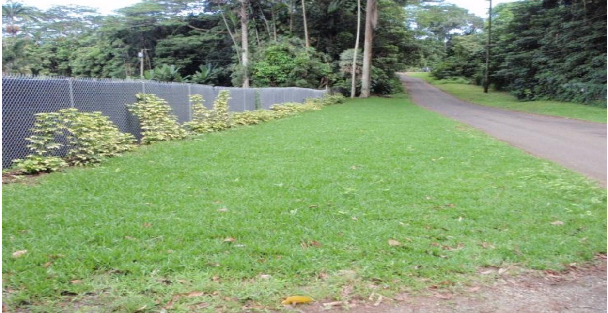
Figure 12: Roadside revegetated to reduce rill erosion during frequent heavy rains in Waimanalo.
